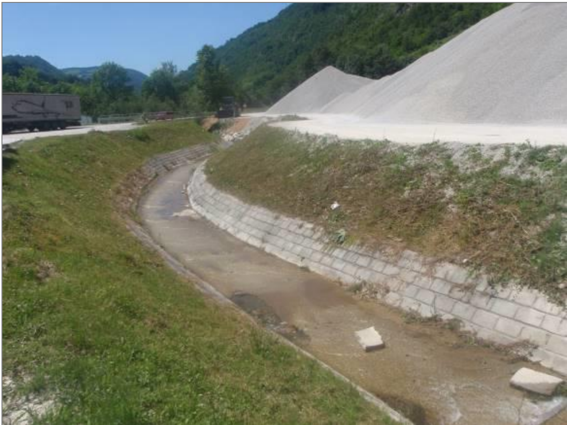
Picture 7 - Regulated river bed of Kozlica river in the area of the quarry
