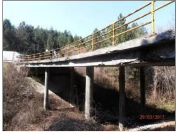
Picture 40 - Bridge over stream (Mrcica bridge)
