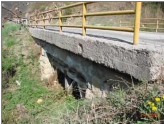
Picture 37 - Bridge over Brdski stream
