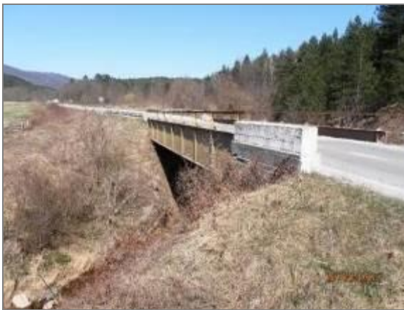
Picture 41 - Bridge over stream in Markovici
