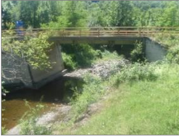
Picture 39 - Bridge over Bukovska river in Bacevci
