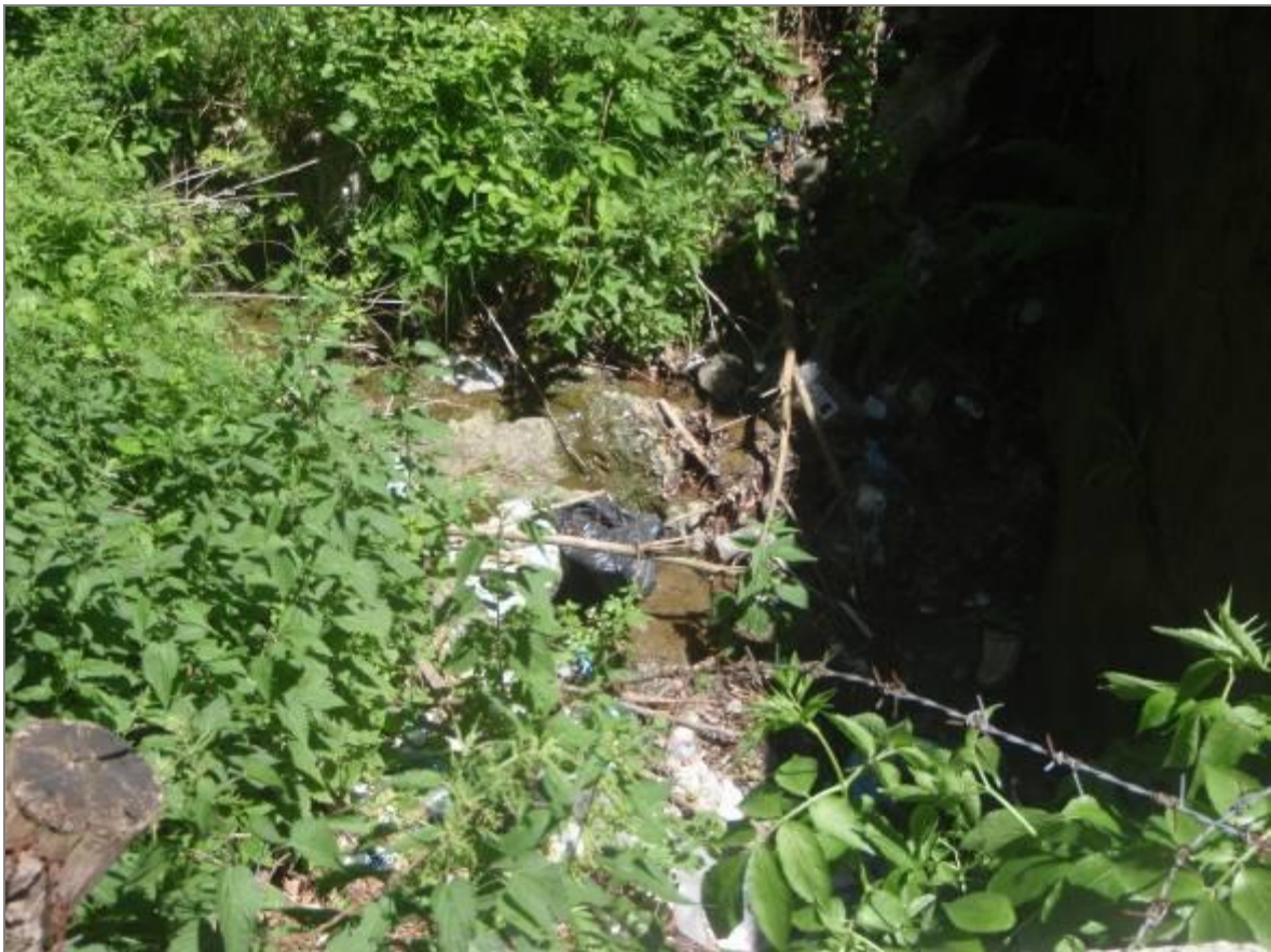
Picture 13 - Culvert covered with vegetation and waste
