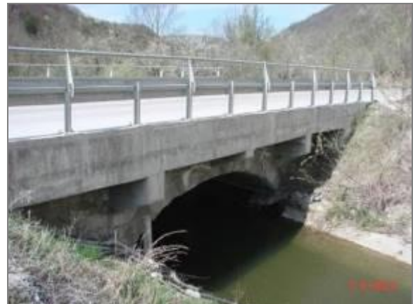
Picture 38 - Bridge over Kozlica river
