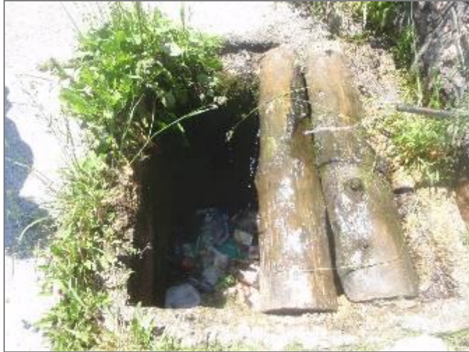
Picture 16 - Garbage in the drain
