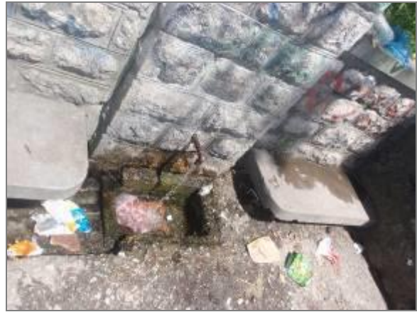
Picture 18 - Garbage around the fountain
