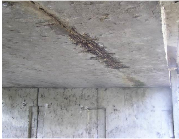
Leakage through the first and the second support
