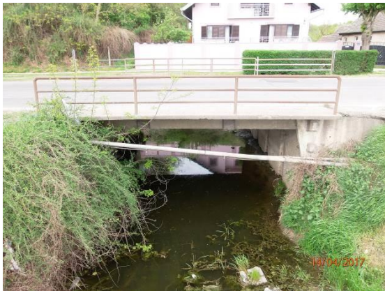
Figure 4 Existing bridge at the road chainage km 63+735
