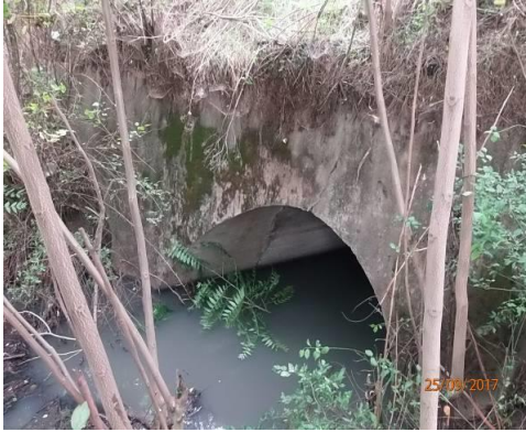
Figure 6 Solid-headed culvert at km 67+845
