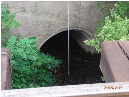
Figure 7 Culvert at km 72+725
