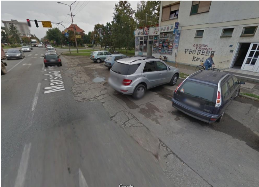
Figure 16. Existing state of the carriageway – different pavement type
