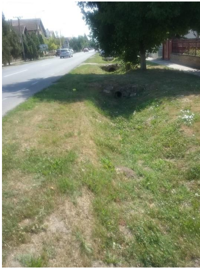
Figure 3 Existing open canal that gravitate to Great Backa Canal
