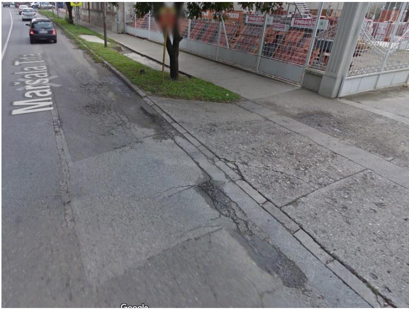
Figure 15. Example of damage of the road section
