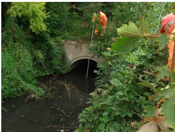
Figure 5 Tubing \phi 2000mm at km 66+925
