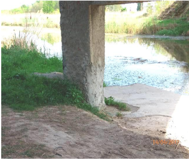
Figure 18 repair of the bottom part of the pier
