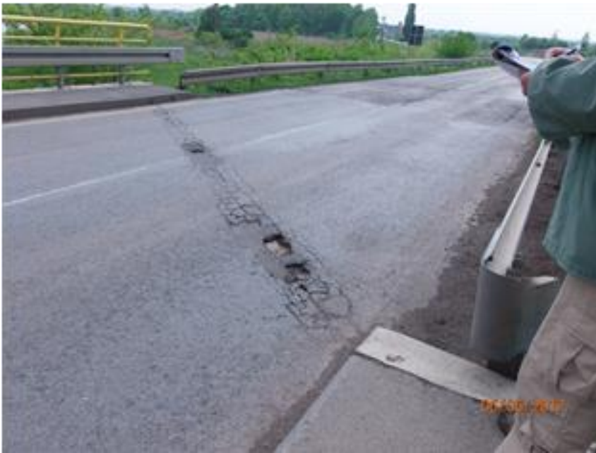
Figure 17. Crack in the pavement at the end of the structure
