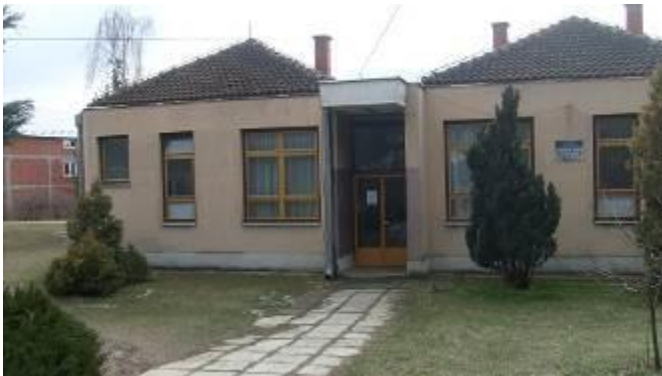
Figure 3.2 - Primary school "Jastrebacki partizani" in Merosina
