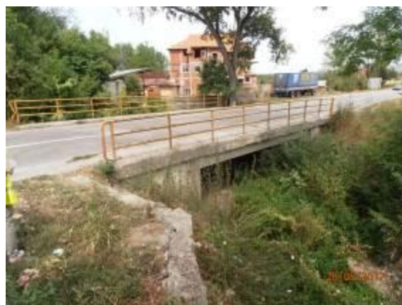
Figure 3.14 - Bridge over the Jugbogdanovacka River
