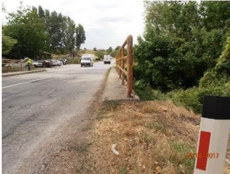
Figure 1.6 – bridge over the Jugbogdanovacka River
