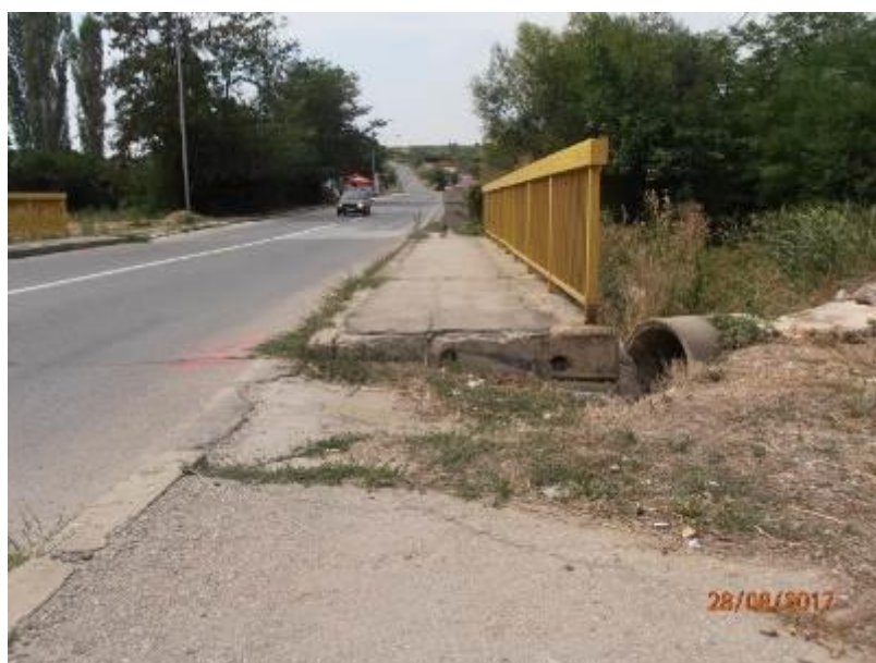
Figure 1.5 – bridge over the Krajkovacka River
