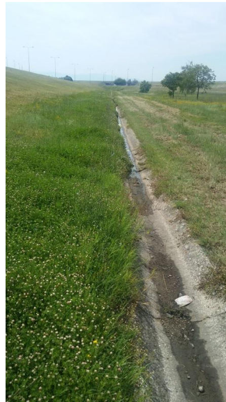
Figure 4. Ditch with concrete cover
