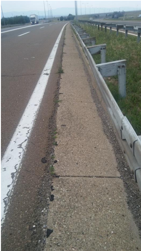
Figure 11. Concrete curb along the central reserve
