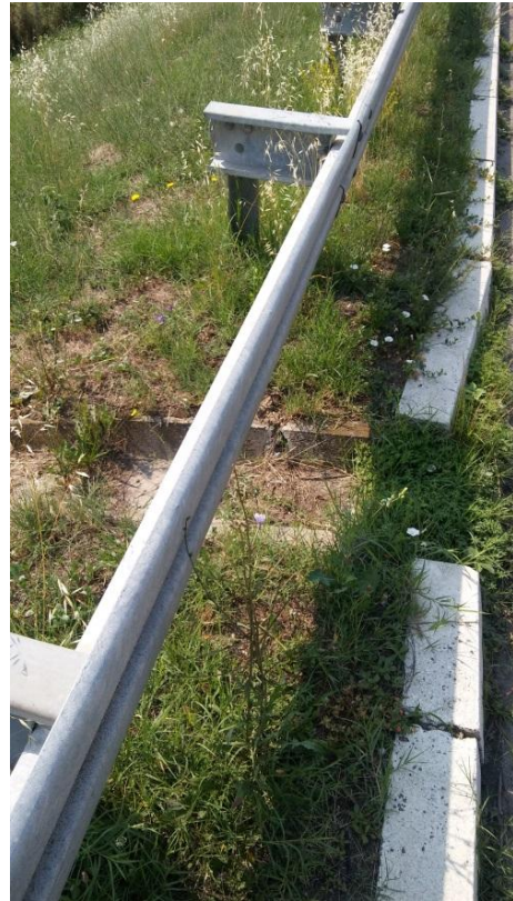
Figure 8. The outflow from the pavement into the concrete gutters
