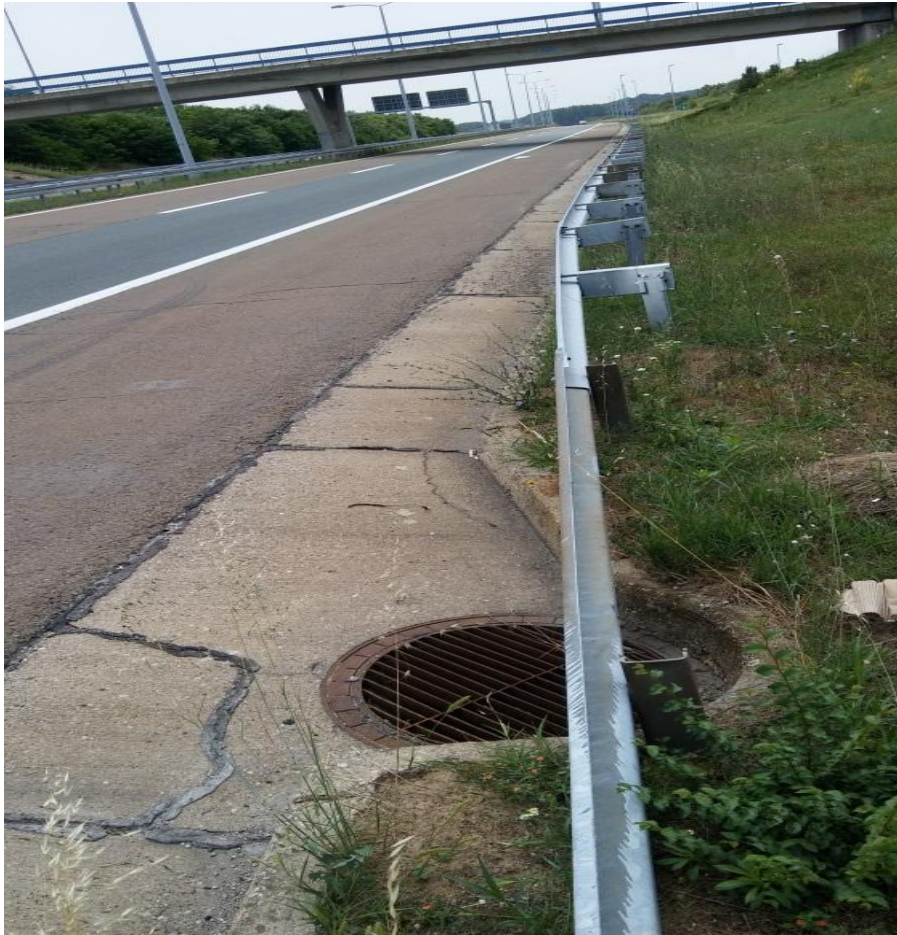
Figure 13. The inflow curb in the manhole over the drain cover on the right edge of the pavement (interchange Merosina)
