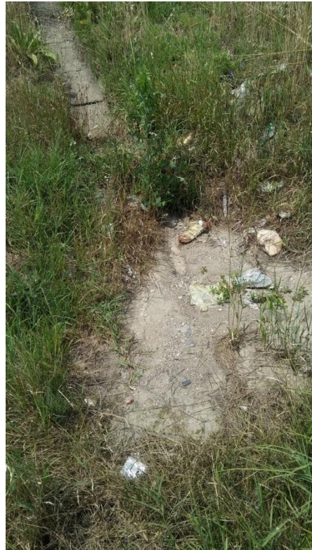
Figure 10. The outflow of drainage canal with concrete gutters
