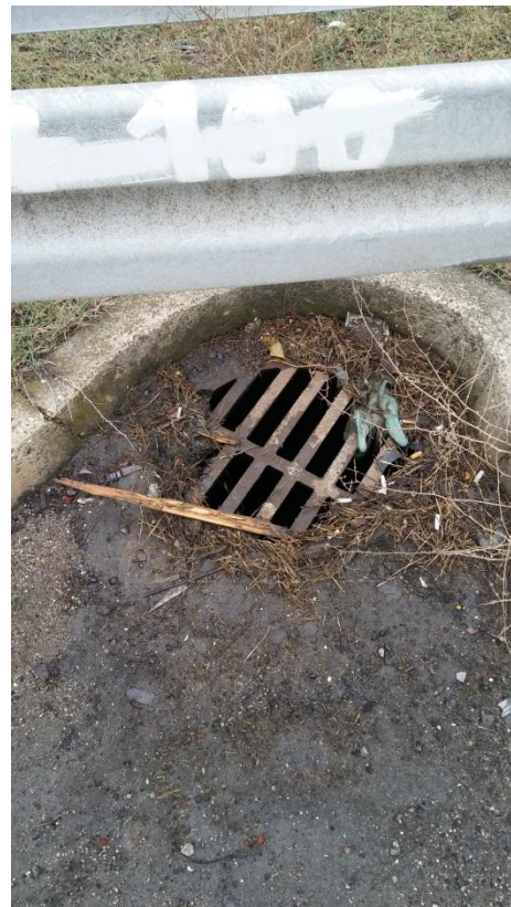
Figure 12. The inflow curb in the manhole over the drain covers
