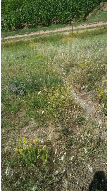
Figure 9. Drainage canal with concrete gutters
