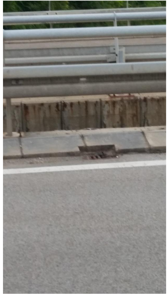
Figure 15. The bridge drains
