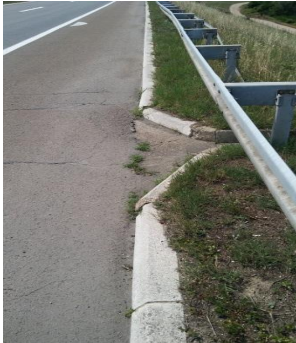
Figure 17. Drainage with a curb system and drainage concrete gutters in front and behind the bridge
