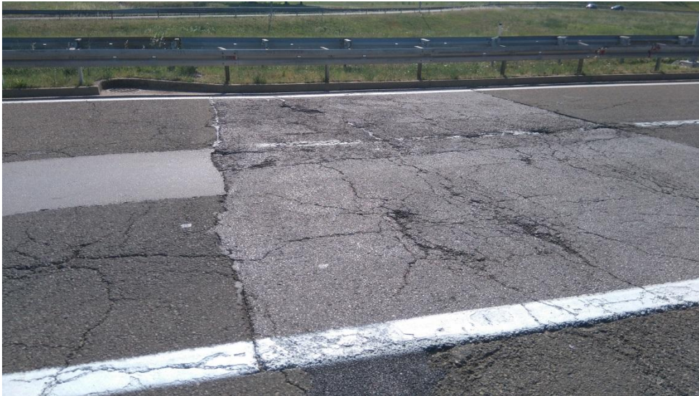
Figure 22. Example of damage of the road section
