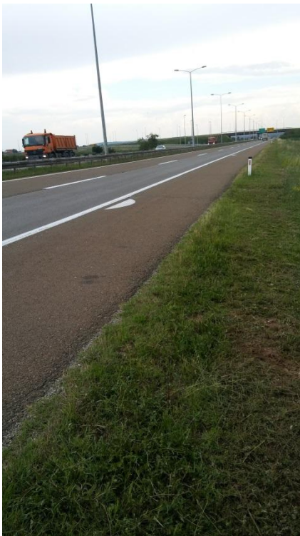
Figure 5. The maintained shoulder
