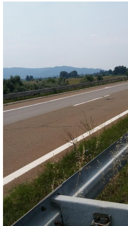
Figure 6. The shoulder overgrown with grass
