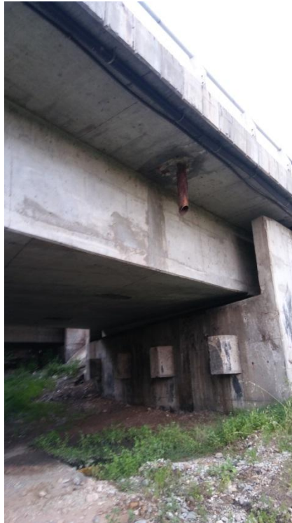
Figure 16. The bridge drains
