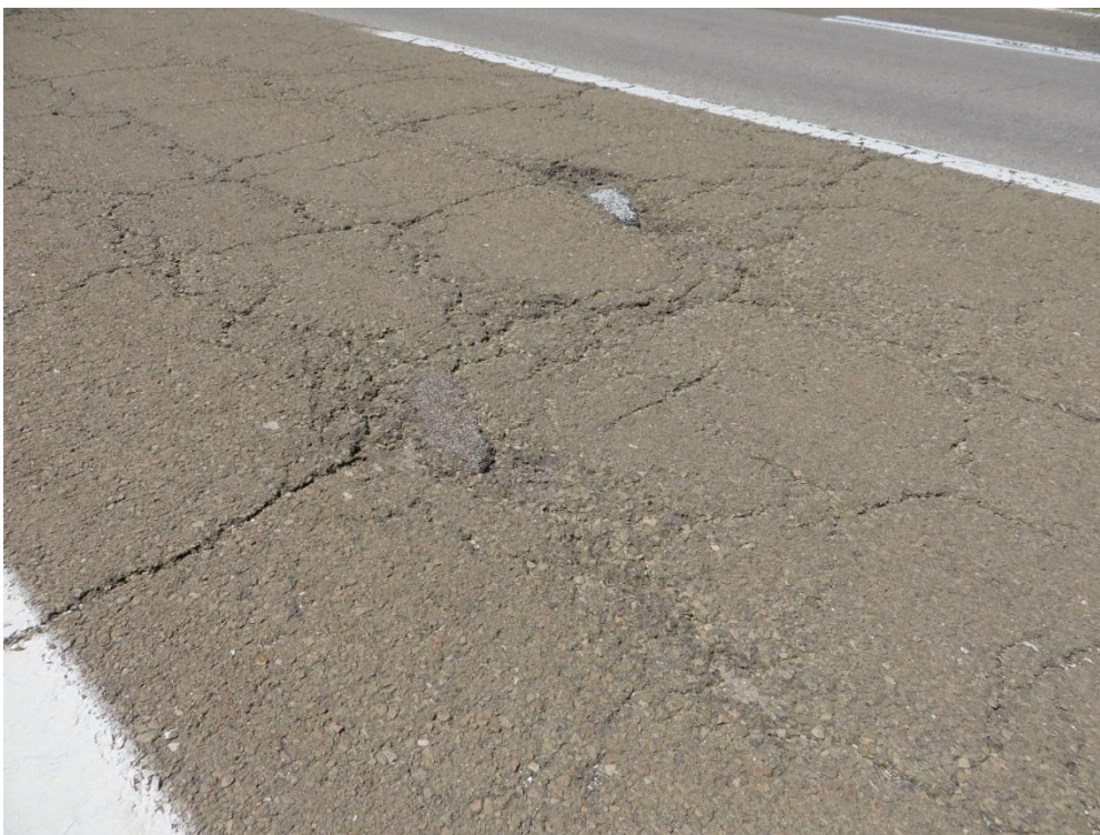
Figure 23. Example of damage of the road section
