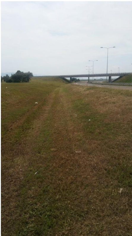
Figure 3. Ditch (drainage canal)
