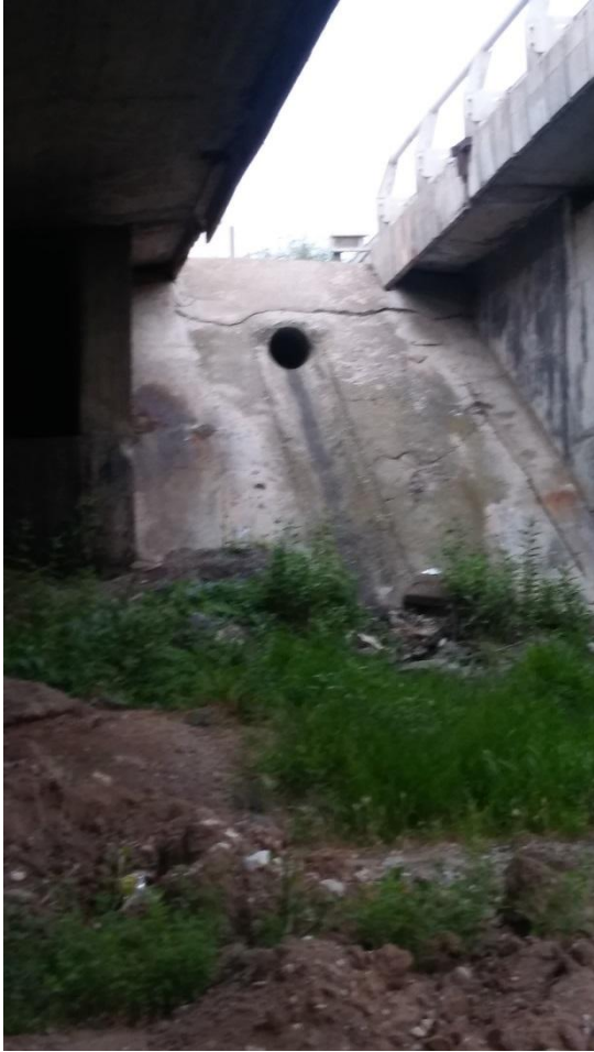
Figure 14. The outflow of the pipeline system down at concrete drainage surface
