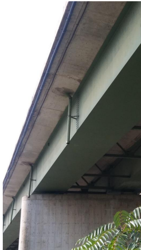
Figure 18 and 19. The bridge drains
