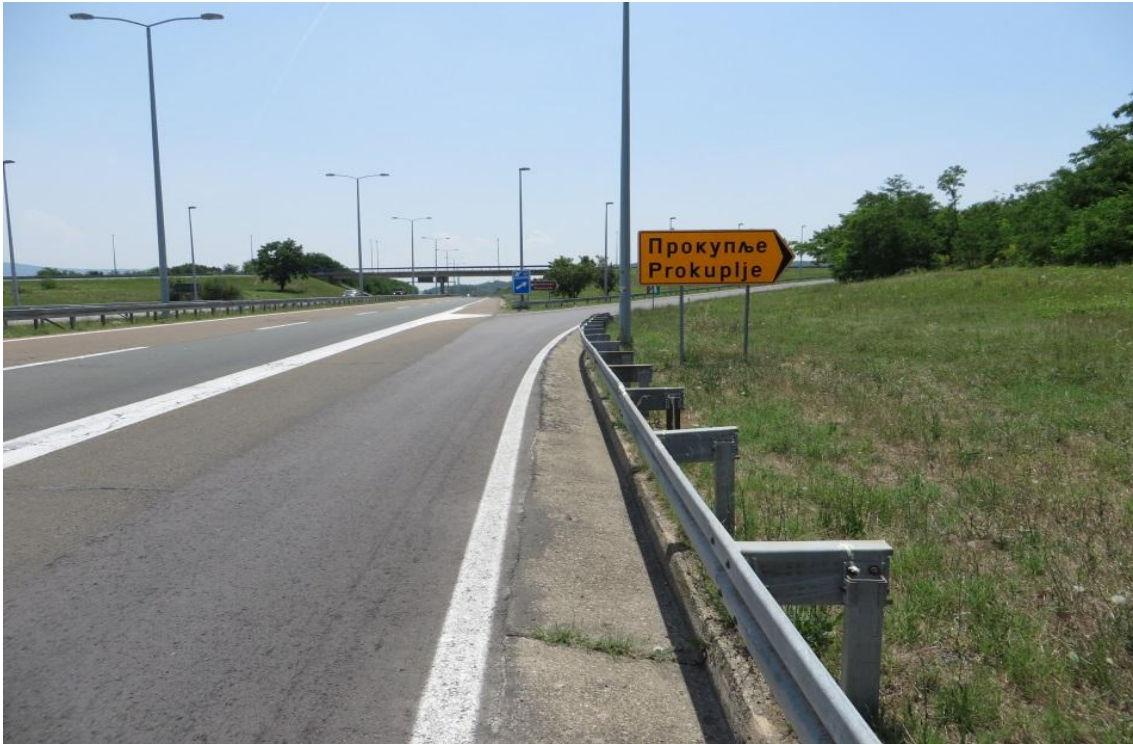
Figure 2. The end of the road section – interchange Merosina
