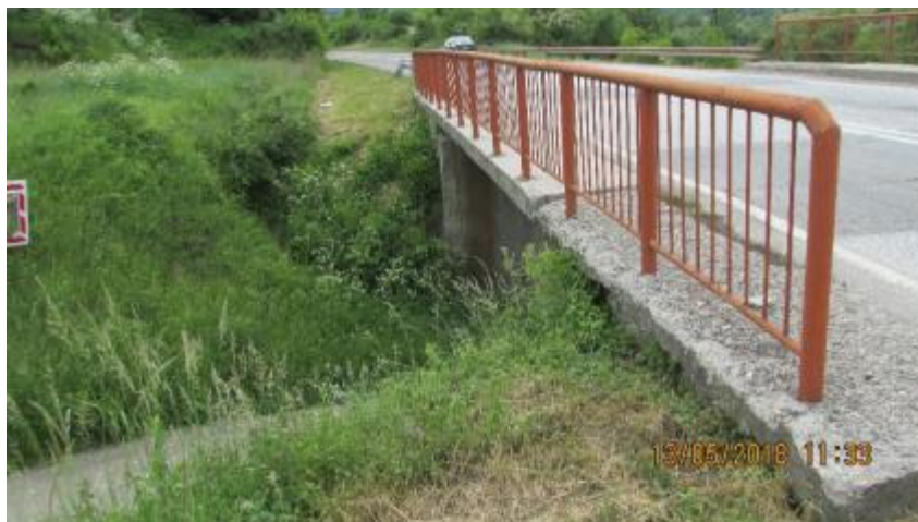
Figure 28. The Bridge over Local Road at km 241+323
