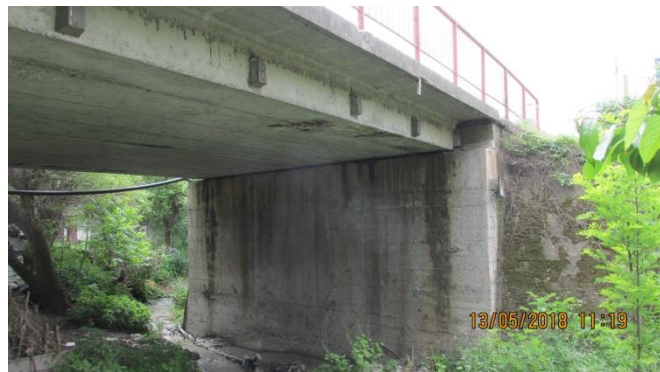
Figure 22. The Bridge over the Bisina River
