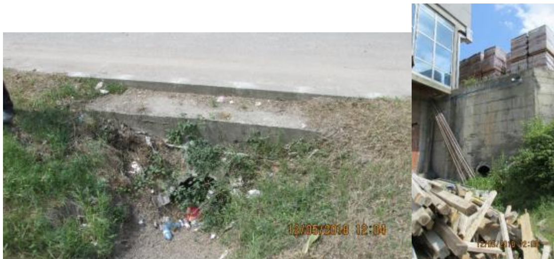
Figure 26. The pipe culvert at km 249+784, outlet and inlet structure of the culvert
