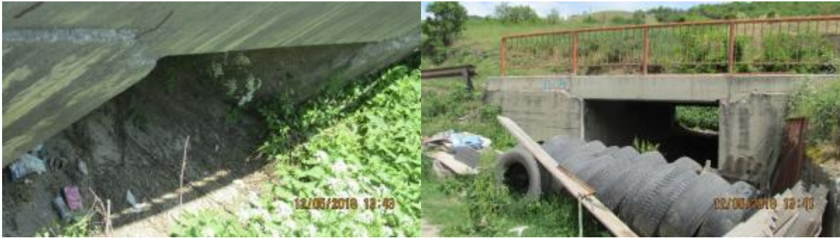
Figure 27. The slab culvert at km 250+790, outlet and inlet structure of the culvert
