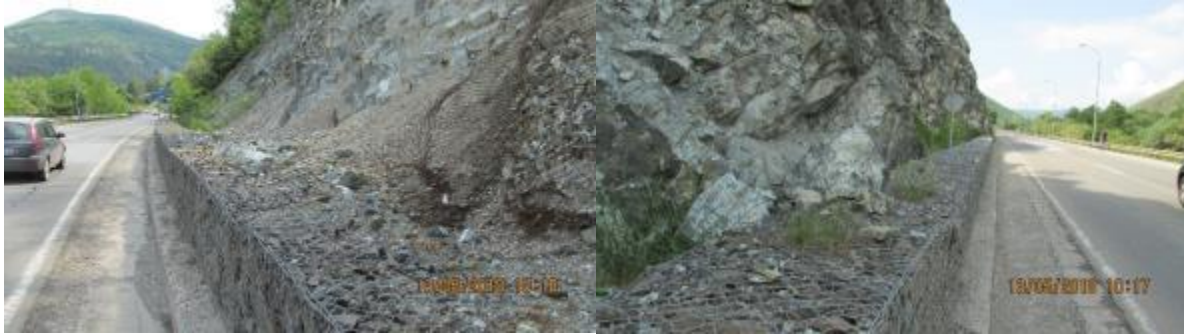
Figure 9. Gabions on the subject section
