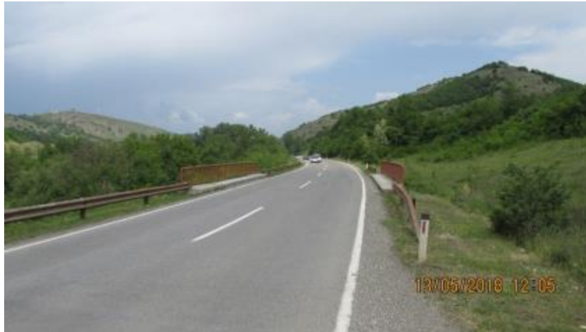
Figure 29. The Bridge over Local Road at km 244+058
