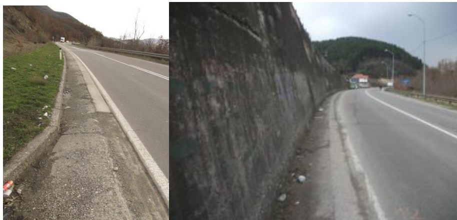
Figure 13. Gutters on the subject section
