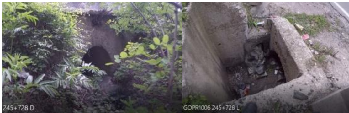
Figure 25. The arched culvert at km 245+728, outlet and inlet structure of the culvert
