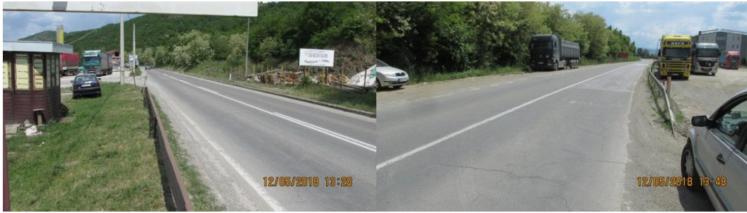
Figure 19. Parking lots for trucks in the road zone
