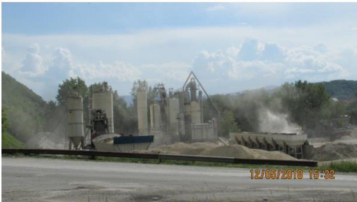
Figure 18. AD Novi Pazar Put from km 252+560 to km 252+900 on the right side of the subject road section
