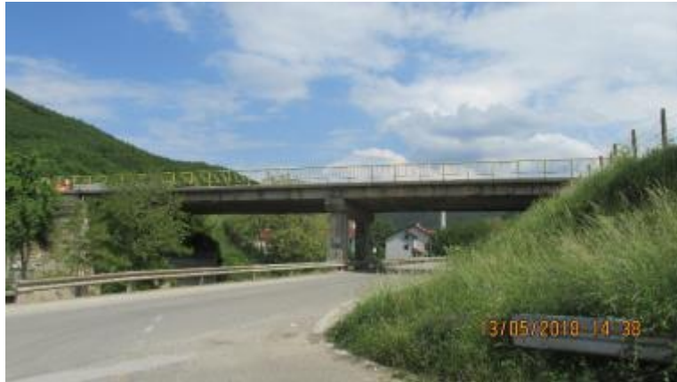
Figure 24. The bridge over the Banjska River and road
