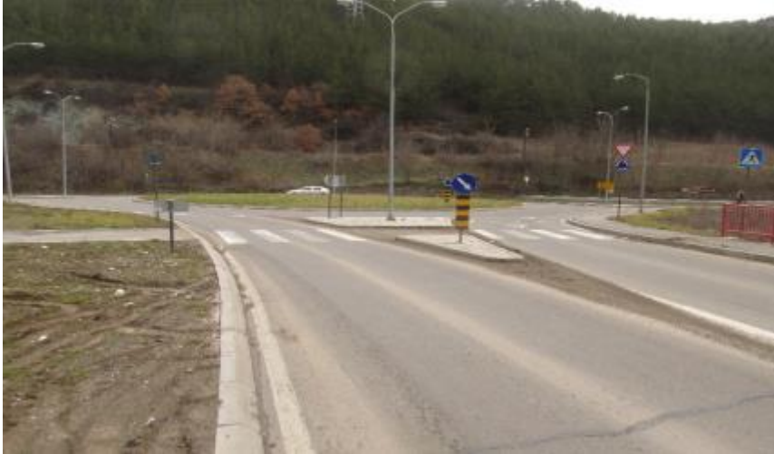
Figure 4. The beginning of the subject road section approximately at km 236+020
