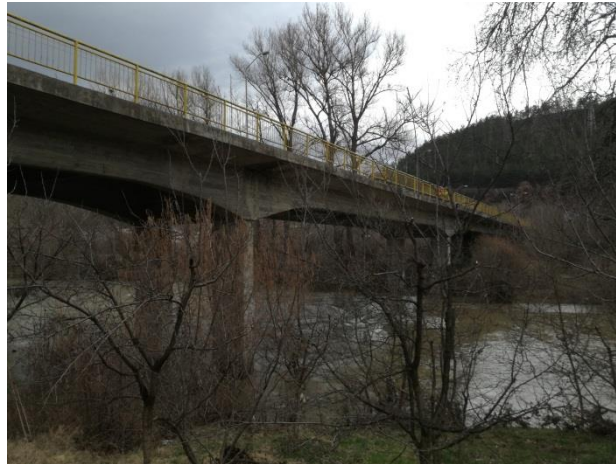
Figure 21. The Bridge over the Ibar River
