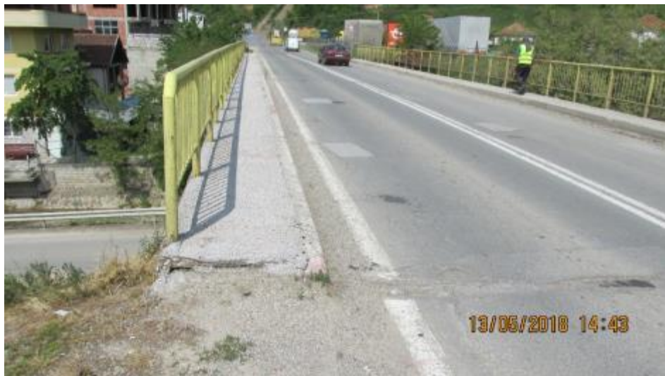
Figure 5. The end of the subject road section approximately at km 253+891
