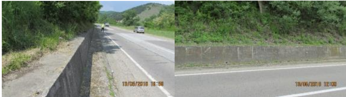
Figure 10. Abutment walls on the subject section
