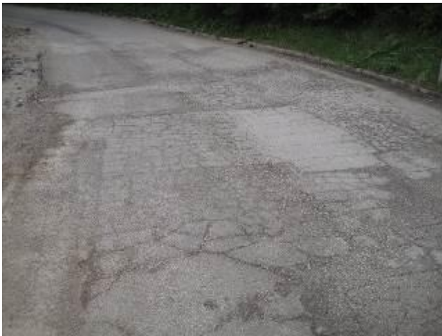
Figures 31, 32 and 33: Example types of damage on the road section
