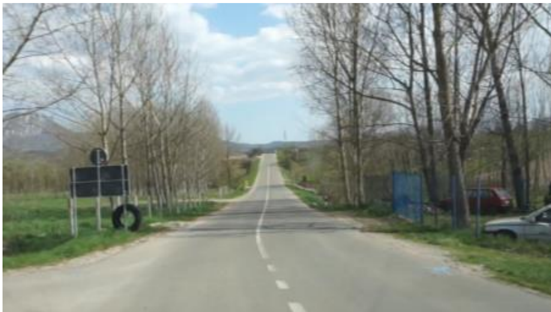
Figure 1. The beginning of the road section – km 25+866
