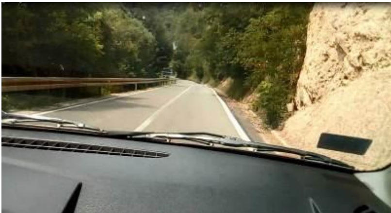
Figure 5: The gutter along the right side of the pavement
