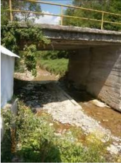
Figure 10: The bridge over the Dolska Valley
