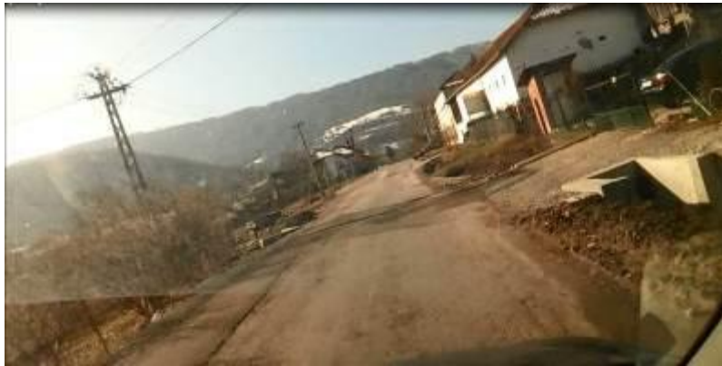
Figure 4: Inlet reinforced-concrete head of the culvert
