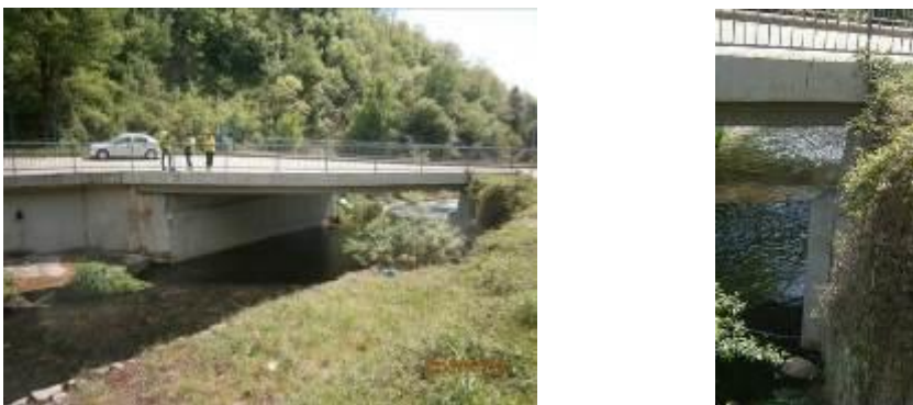
Figure 7 and 8: The bridge over the Luznica River (Intersection no. 2)
