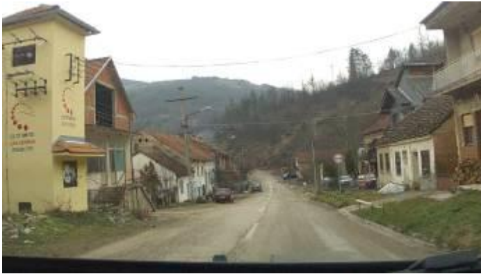
Figure 26: The existing bus stop - Ljuberadja at km 31+028.00
