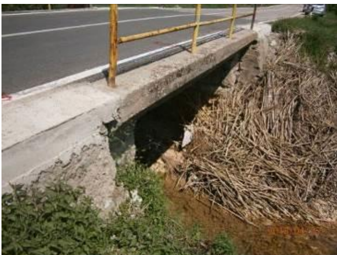
Figure 9: The box culvert over the Linovstica River
