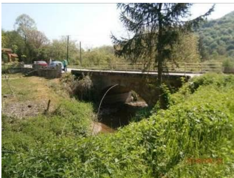
Figure 15: The bridge over the Rdjavica River (Intersection no. 9)
