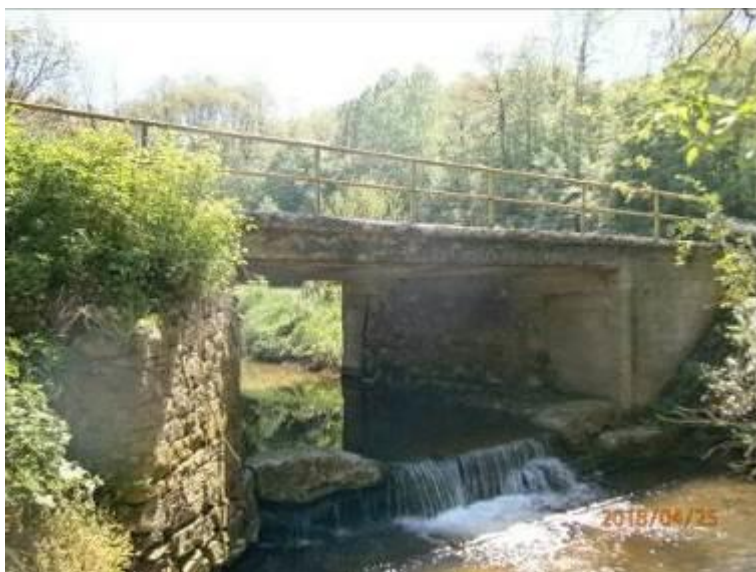
Figure 14: The bridge over the Rdjavica River (Intersection no. 8)
