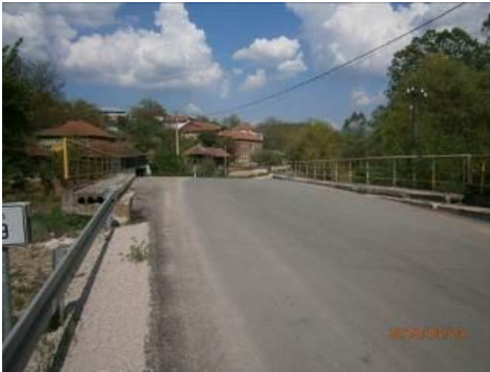
Figure 6: Access to the bridge over the Luznica River (Intersection no. 1)
