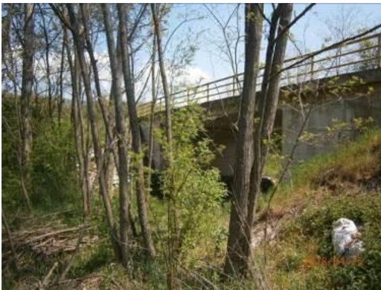
Figure 13: The bridge over the Rdjavica River (Intersection no. 7)
