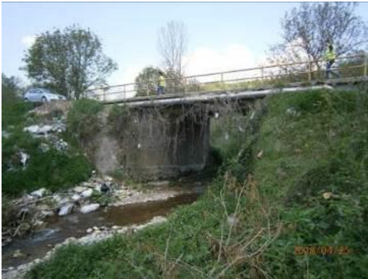
Figure 12: The bridge over the Jablanica River
