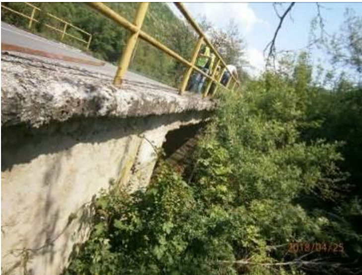
Figure 11: The box culvert over the Brestovdolski Creek
