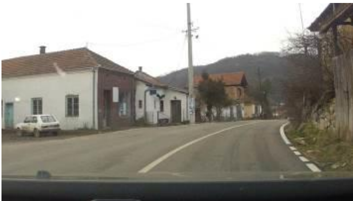
Figure 27: The existing bus stop - Grncar at km 35+078.00
