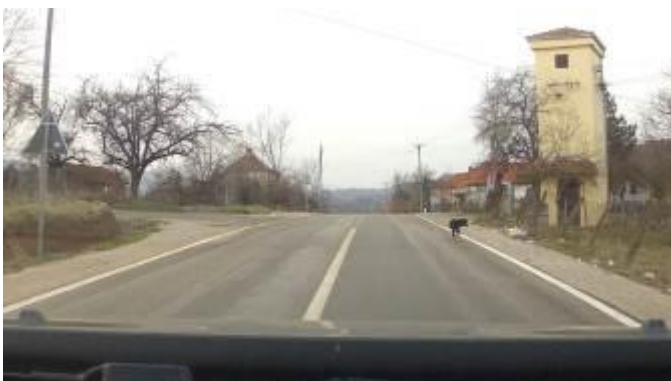
Figure 29: The existing bus stop - Modra Stena at km 39+428.00
