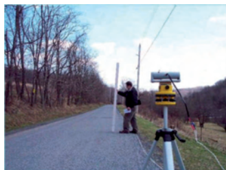
Висински поожј, (20-25 m 1 ) (Leveling position of layer)
