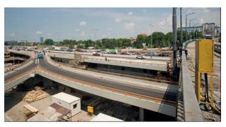
its structure. One, if not the most interesting thing are boxes within the bridge base, at the height of 12m. Most workers perform their work in these boxes although their height is only 1.20m. Gazela bridge consists of 31 parts and each of them hides a team of builders.
