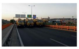
In the night between 11 and 12 August 2012, another load testing of main span of the Gazela bridge, which is integral part of Rehabilitation Project according to the Standard SRPS U.M1.046 – Bridge load testing was performed.
