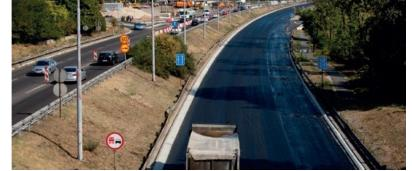
the existing curbs is foreseen, existing asphalt is being replaced by base course – base BNS and SMA wearing course or road surface. In addition to the basic works, there is ongoing repair of damaged elements of the drainage system
