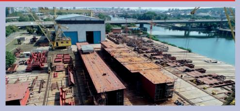
4,900 tons of steel were purchased and processed for the construction of steel bridge - 8 structure over the river, the length of which is to be 586 meters.
