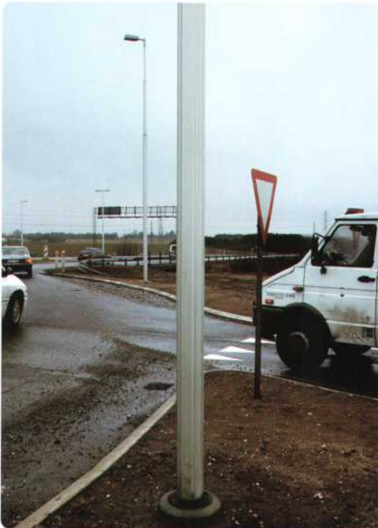
Frangible lighting column.
