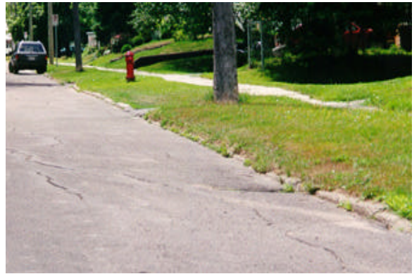
Photo 2. Curbs in disrepair
