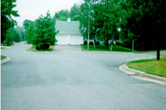
Photo 9. Unsigned confusing alignment
