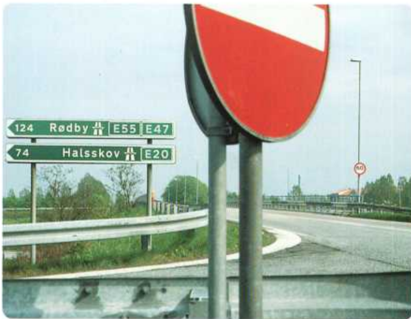
Visibility obscured by road equipment
