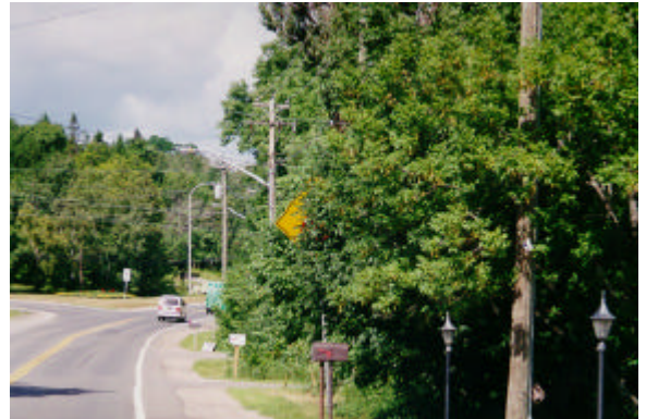
Photo 16. Blocked Stop sign
