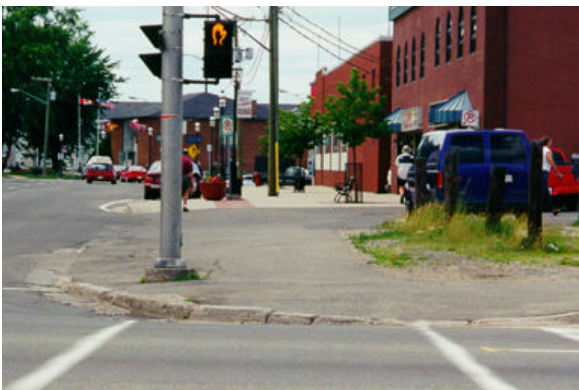
Photo 3. Inadequate curb cut-outs
