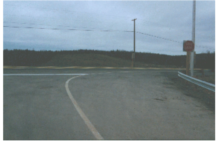
Photo 2: Excessive offset to stop sign (Route 25) off-ramp.
