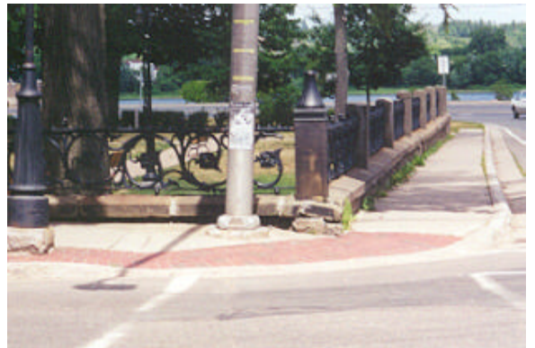
Photo 24. Pole in pedestrian path
