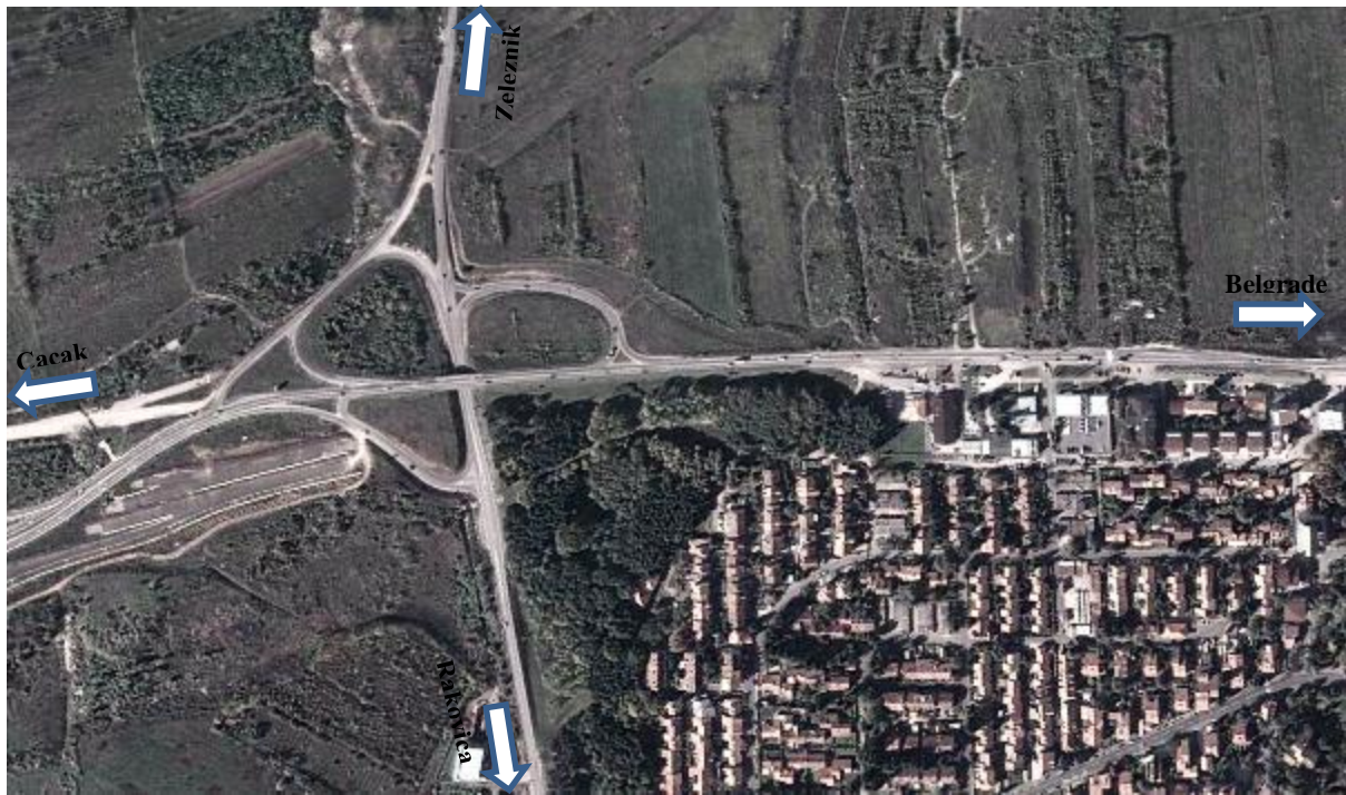
Picture 01: The existing – already constructed “Petlovo Brdo” Interchange
