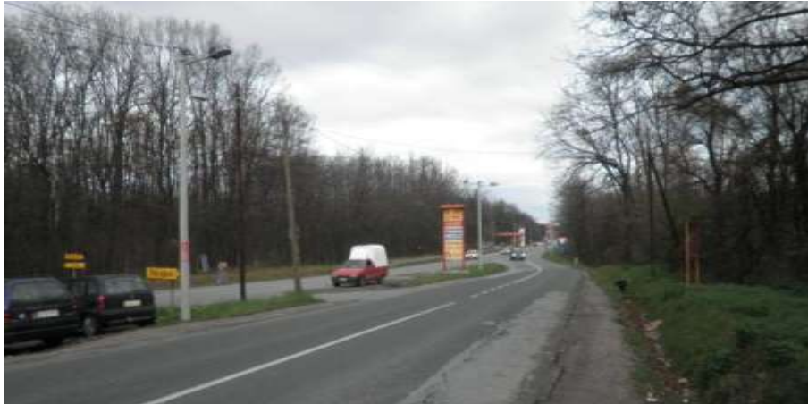
Unsafe design of T-intersection (M-22, Barajevo)
