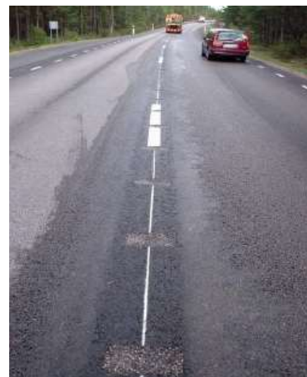
Milled median rumble strips
