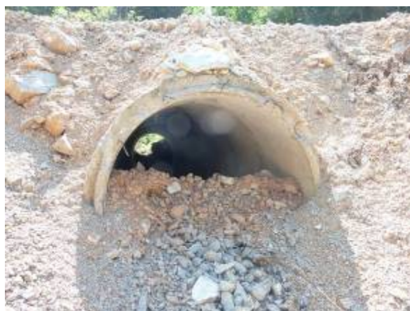
Picture 32. Culvert at 6+041.08 km
