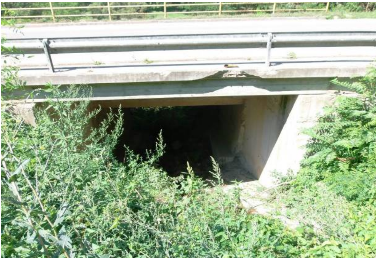
Picture 14. A bridge over the unnamed streambed at 1+800 km
