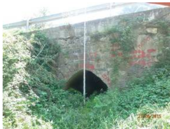
Picture 26. Culvert at 3+356.57 km
