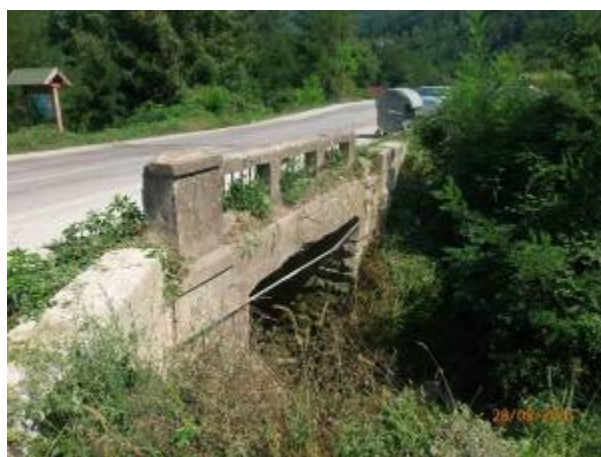
Picture 29. Culvert at 4+074.07 km
