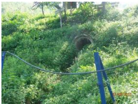
Picture 25. Culvert at 3+299.35 km
