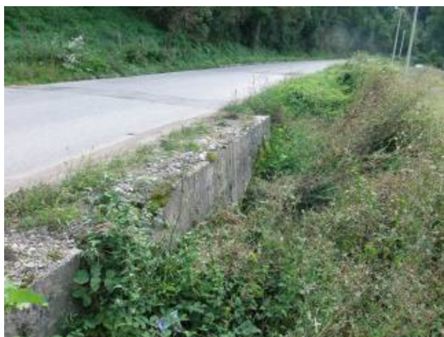
Picture 15. Culvert at 0+180 km
