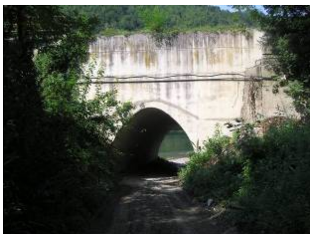
Picture 31. Culvert at 4+488.72 km
