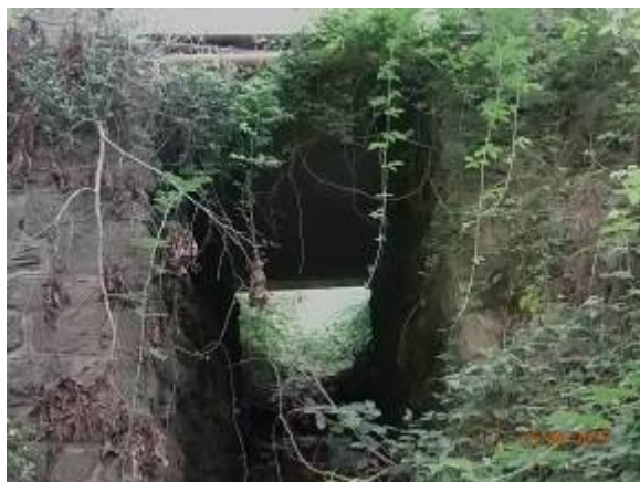
Picture 18. Culvert at 2+038.94 km
