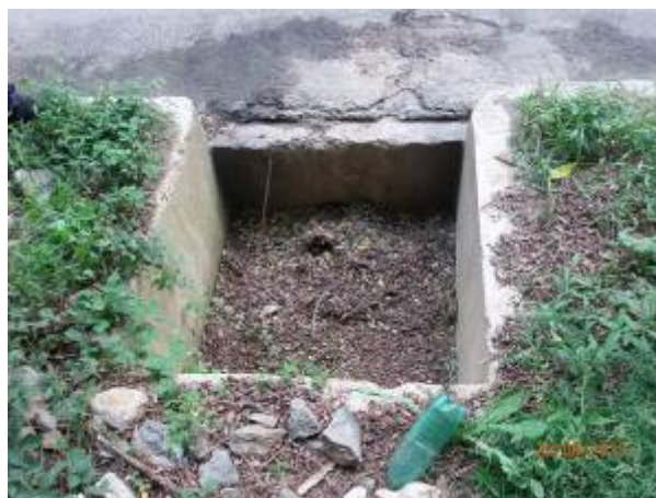
Picture 17. Culvert at 1+838.76 km
