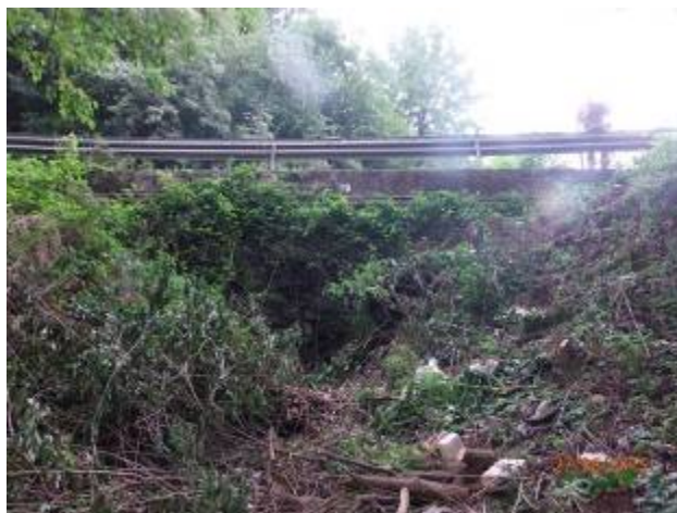
Picture 21. Culvert at 2+394.71 km
