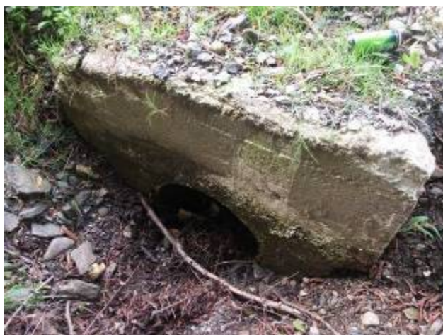
Picture 16. Culvert at 0+446.82 km
