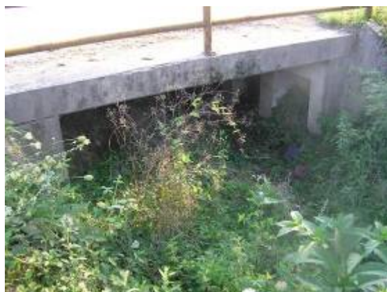
Picture 35. Culvert at 6+885.36 km
