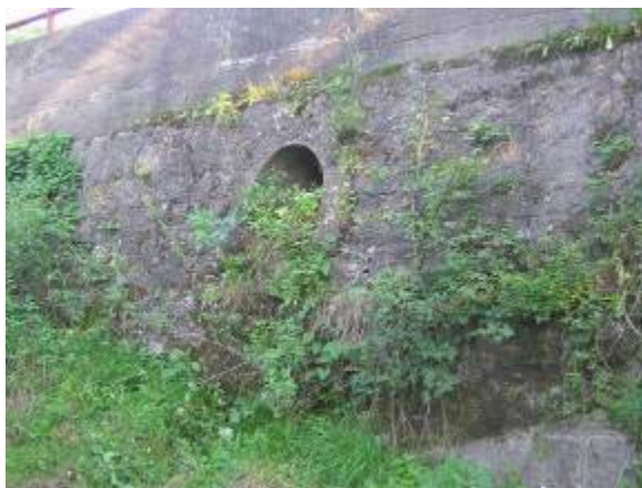
Picture 33. Culvert at 6+597.71 km
