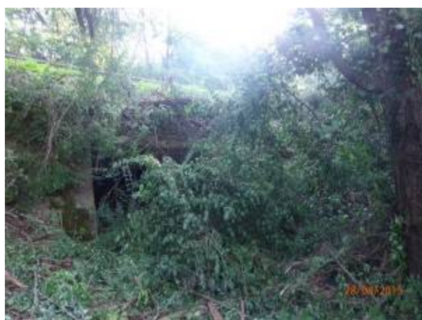
Picture 20. Culvert at 2+268.67 km
