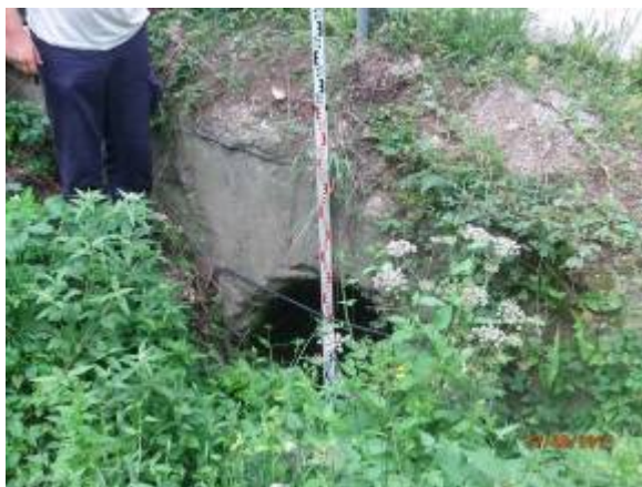
Picture 24. Culvert at 3+137.41 km
