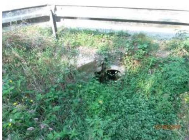
Picture 23. Culvert at 3+002.76 km
