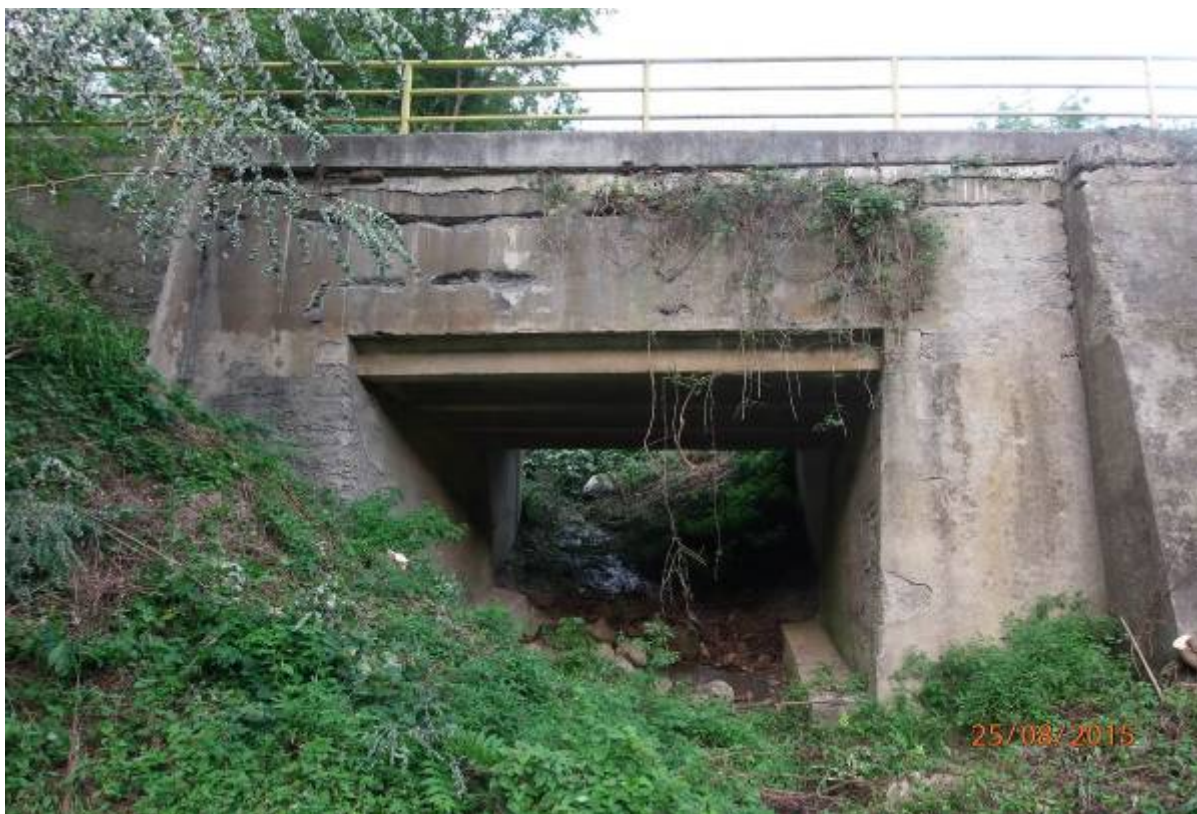
Picture 13. A bridge over the unnamed streambed at 1+800 km
