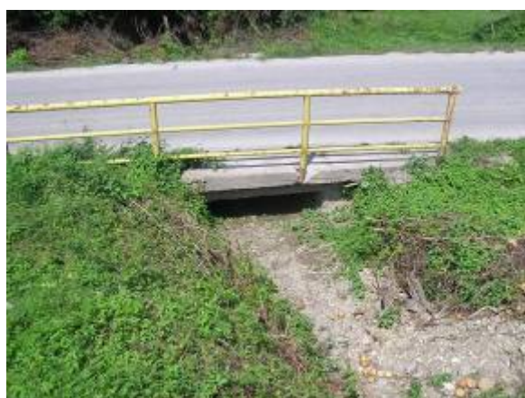
Picture 28. Culvert at 3+847.45 km
