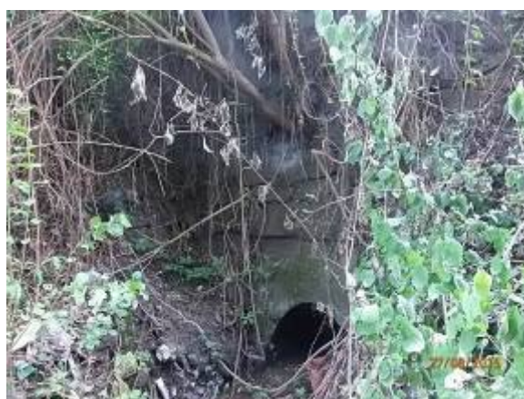
Picture 22. Culvert at 2+670.75 km
