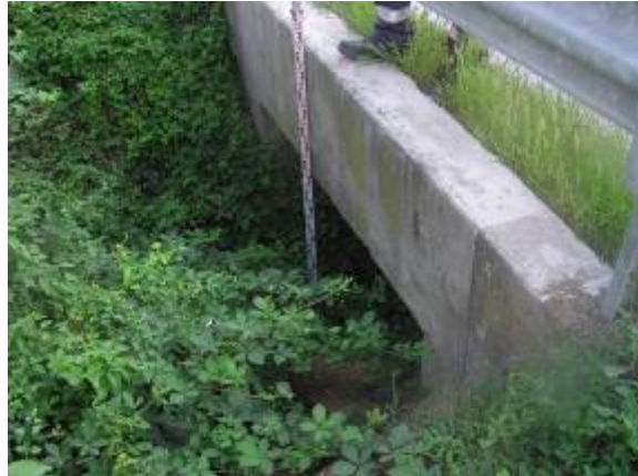
Picture 36. Culvert at 9+369.67 km
