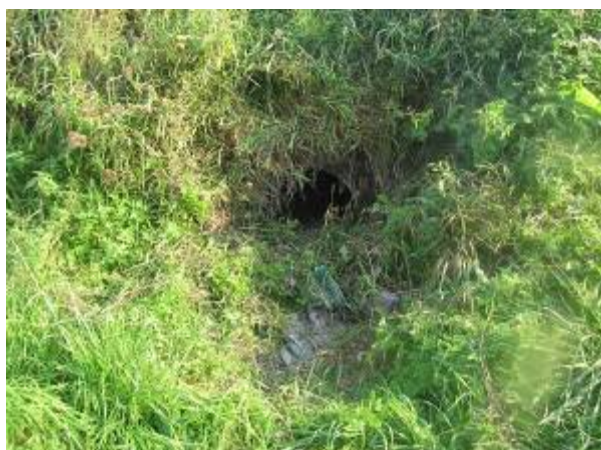
Picture 34. Culvert at 6+765.64 km
