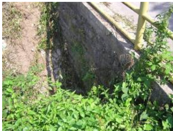
Picture 27. Culvert at 3+669.38 km
