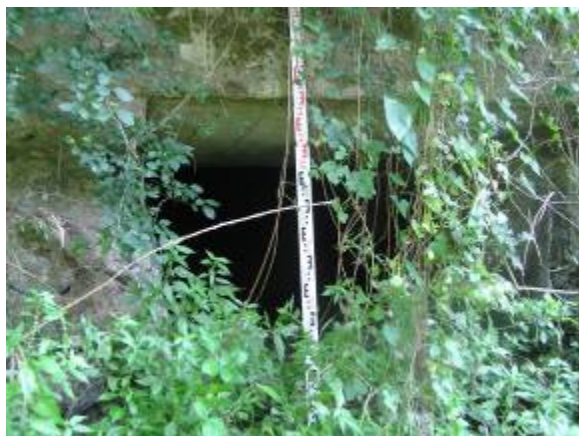
Picture 30. Culvert at 4+375.40 km
