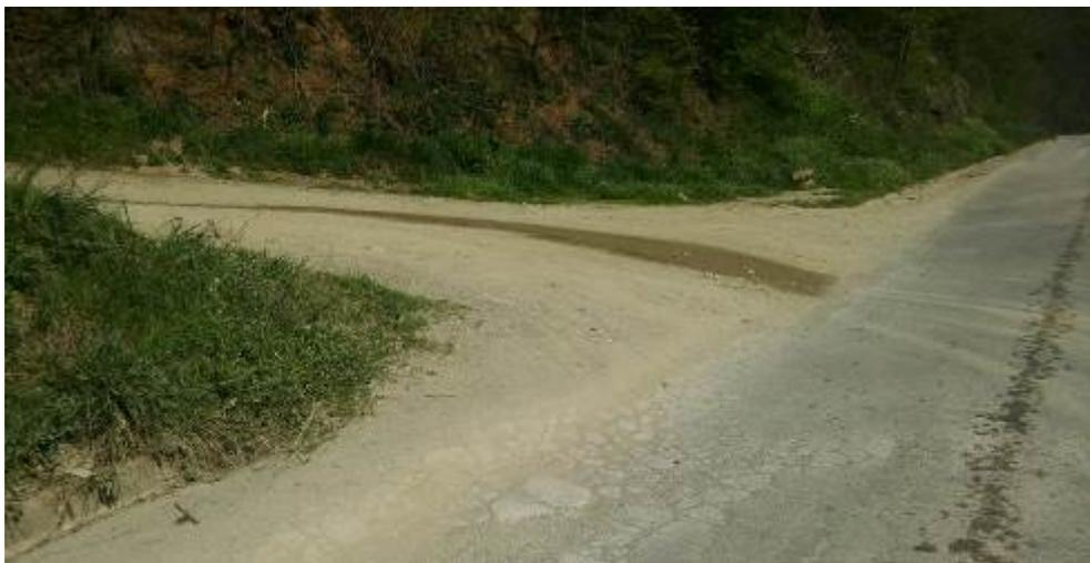
Figure 5. Example of the damage of the section – soil deposit at the road
