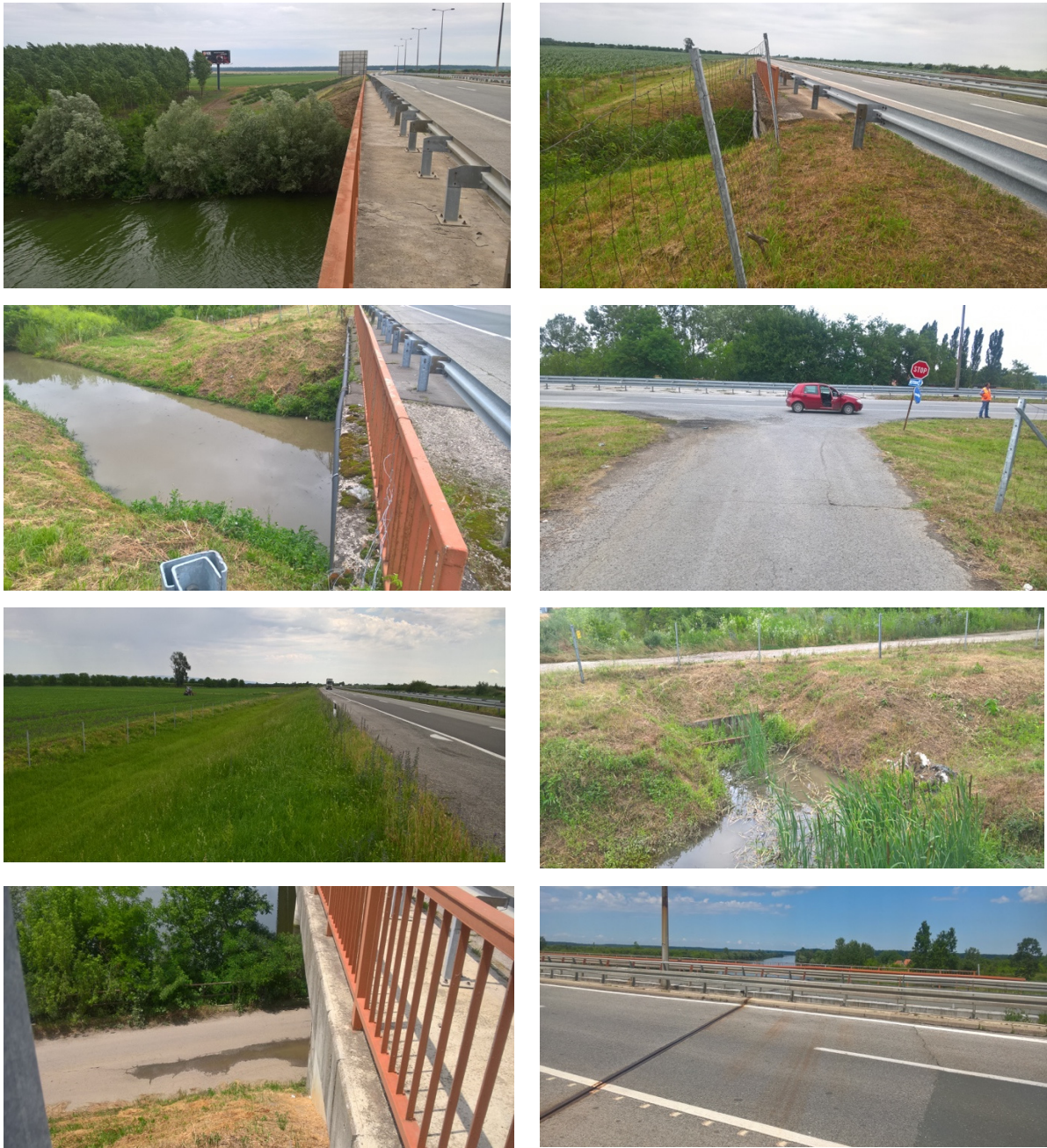
Picture 3. Typical segments along the section
