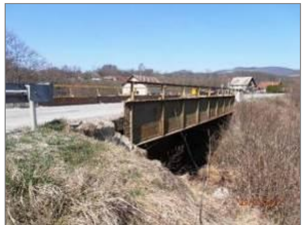
Picture 42 - Bridge over stream at the end of the section
