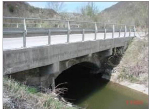
Picture 38 - Bridge over Kozlica river
