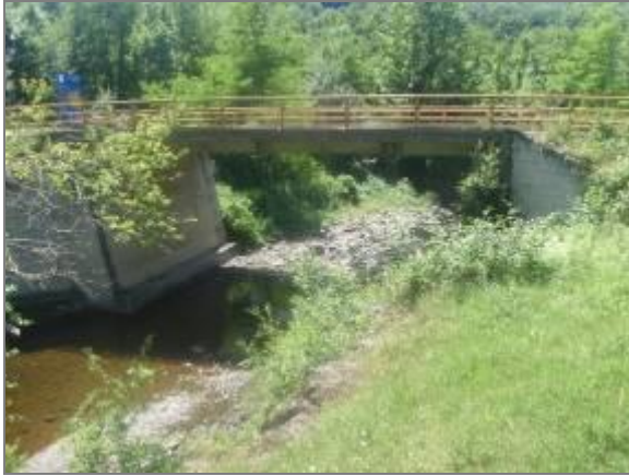
Picture 39 - Bridge over Bukovska river in Bacevci
