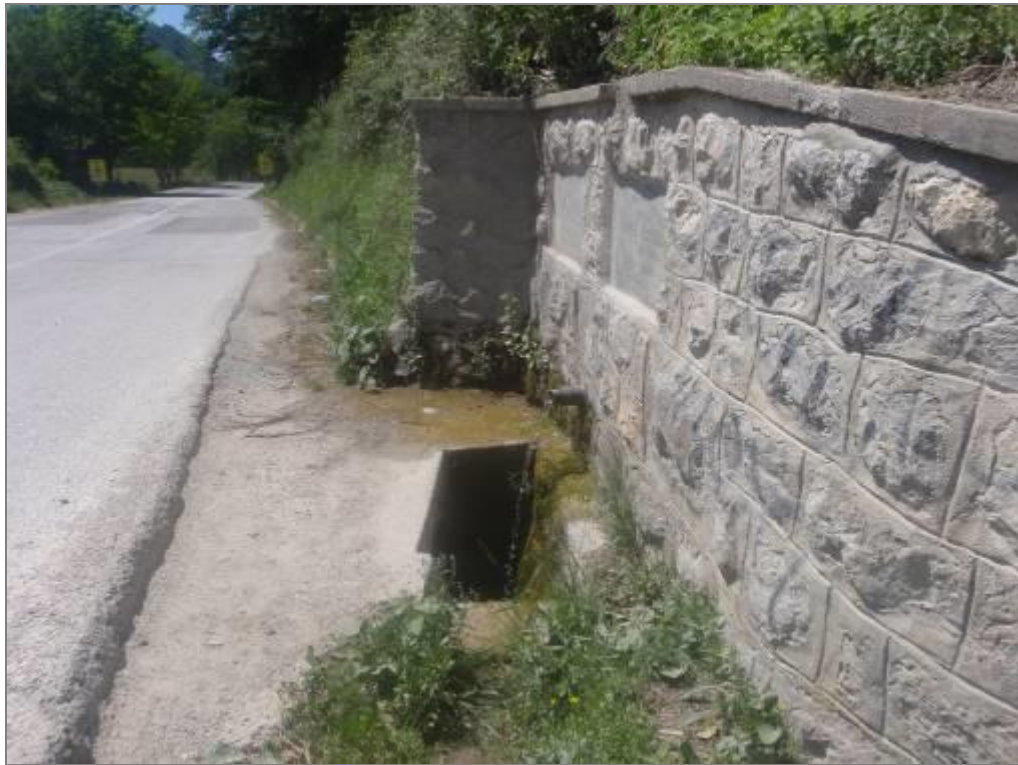
Picture 15 - Fountain at the "Podbukovi" quarry
