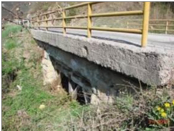
Picture 37 - Bridge over Brdski stream
