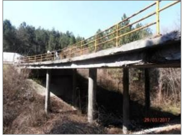
Picture 40 - Bridge over stream (Mrcica bridge)
