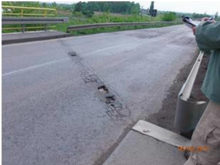
Figure 17. Crack in the pavement at the end of the structure
