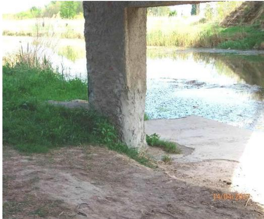
*Figure 18 repair of the bottom part of the pier*
