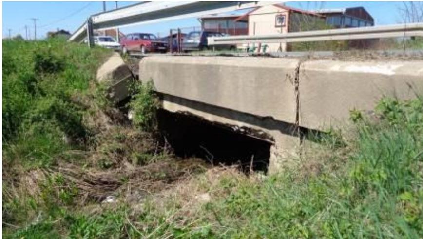
*Picture 18. Box culvert for the occasional torrential watercourse*
