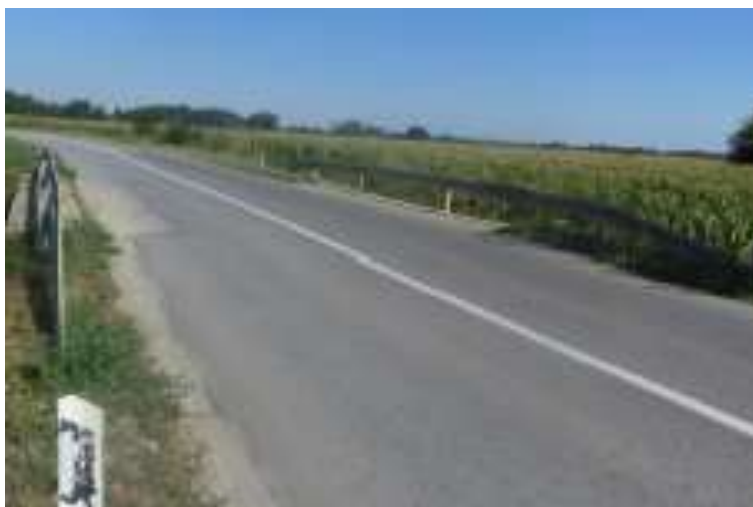
Picture 9. Culvert no.1 on km 190+800.00
