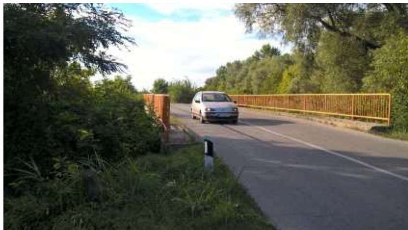
Picture 14. Bridge over Rača River
