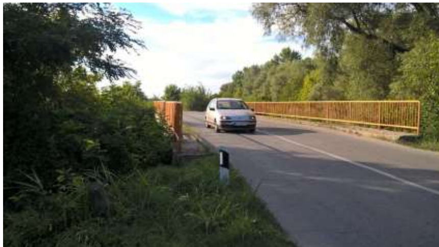
Picture 5. Bridge over Rača River
