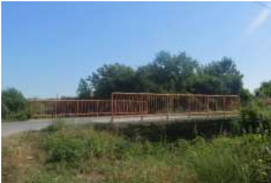
Picture 8. Culvert no. 1 km 190+400.00
