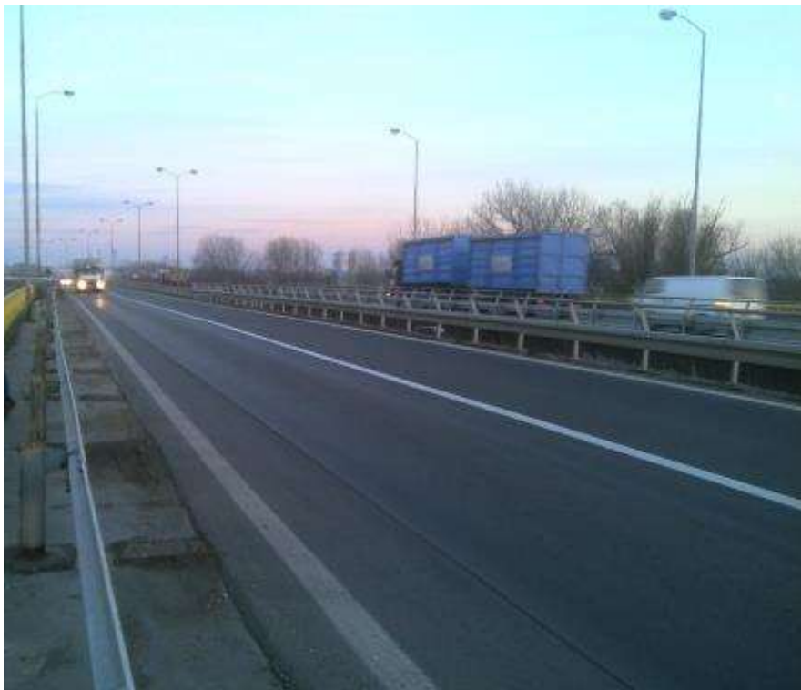
Picture 5. Bridge profile - left lane
