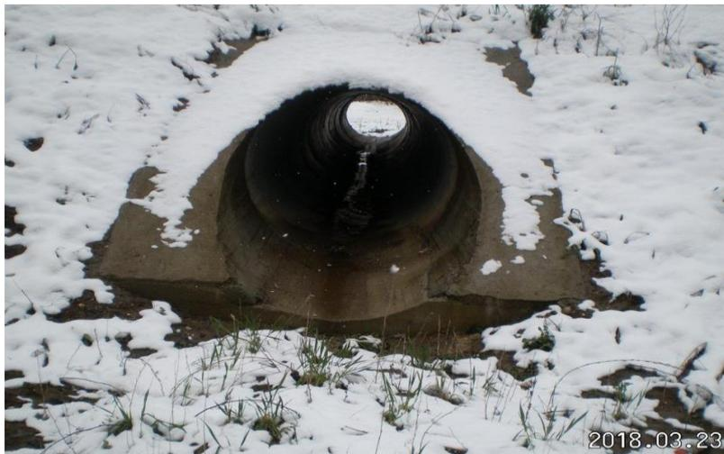
**Picture 13.** Tubular culvert  $\varnothing$  1400 at km 10+337 – no function/ out of order
