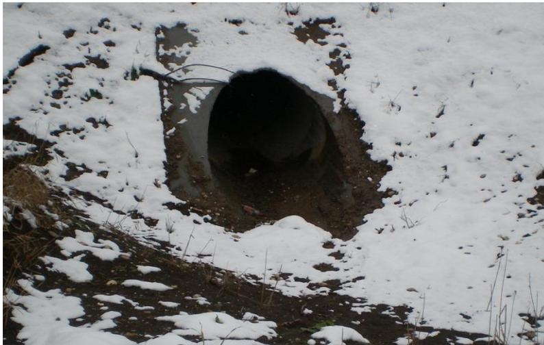
**Picture 12.** Tubular culvert  $\varnothing$  1000 at km 6+358
