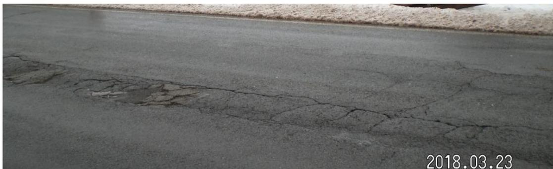
**Picture 37.** The example of damage to the section
