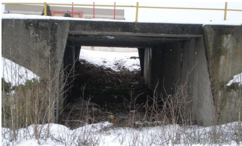
**Picture 14.** Box culvert at km 12+013 – no function/ out of order
