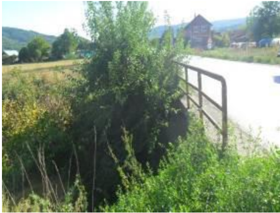
Figure 26. Bridge over the stream in the village of Tulari
