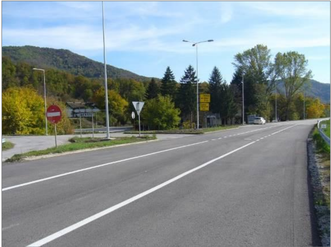
Figure 2. End of the section
