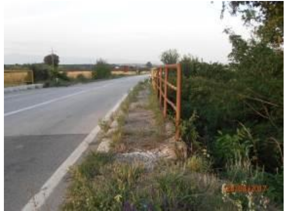
Figure 27. Bridge over the Backa River
