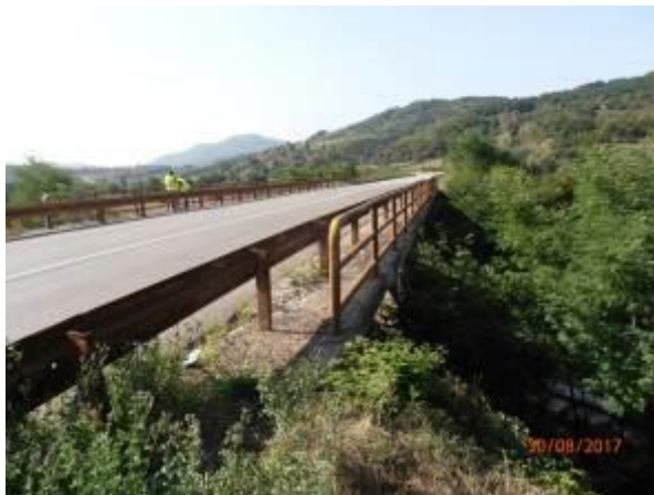
Figure 30. Bridge over the railway
