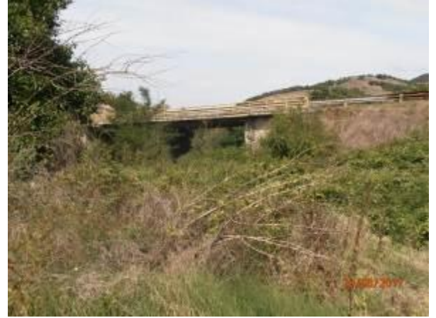
Figure 33. Bridge 2 over the Kosanica River
