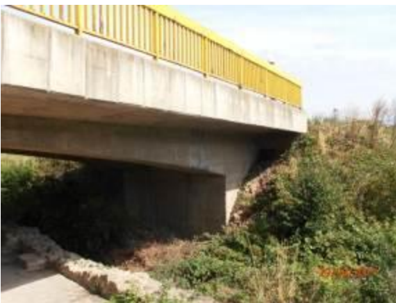
Figure 28. Bridge over the archaeological site
