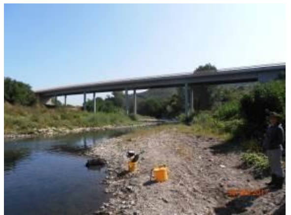
Figure 29. Bridge over the Toplica River
