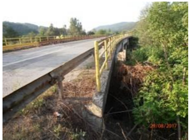
Figure 31. Bridge 1 over the Kosanica River
