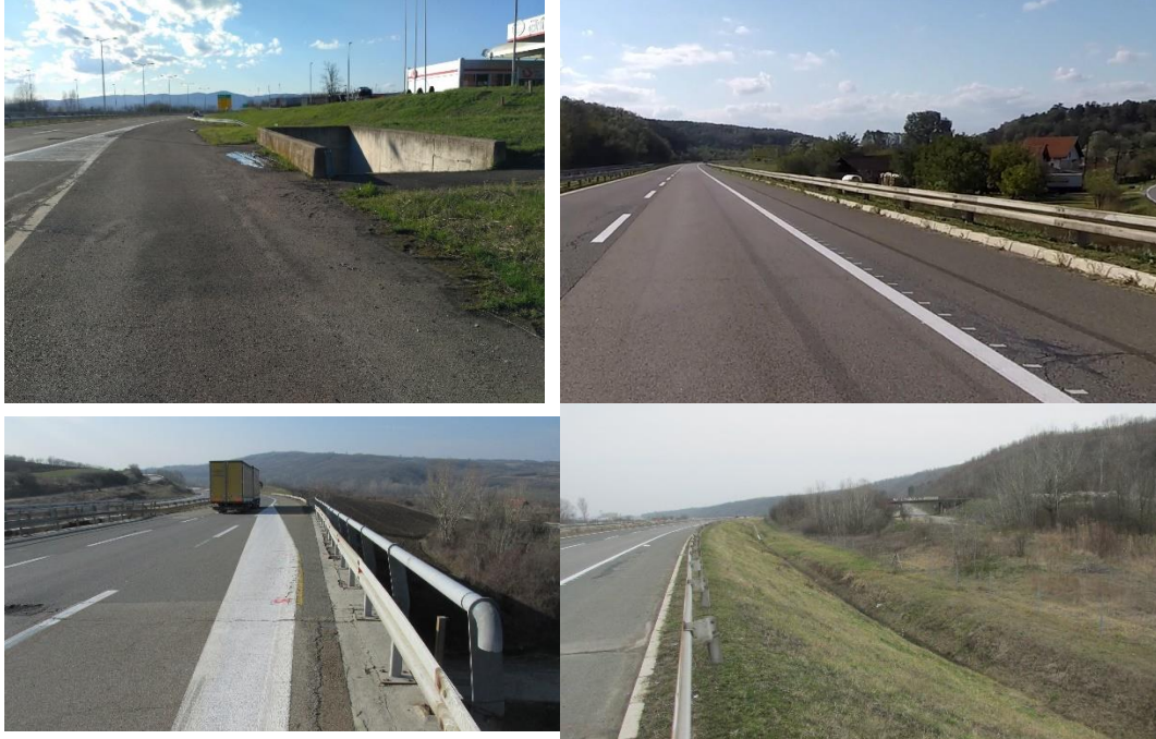
Figure 7. Typical parts of the subject section
