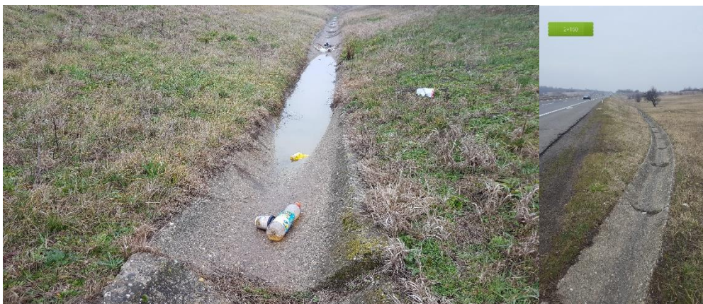
Figure 9. Concrete canals on the subject section
