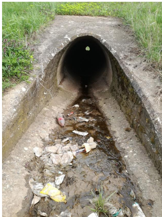
Figure 17. Arched culvert at km 361+767
