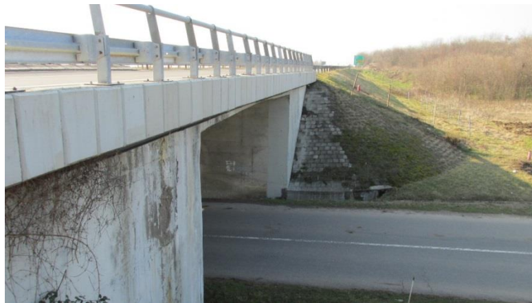
Figure 21. The Bridge over the road 158E at km 373+850
