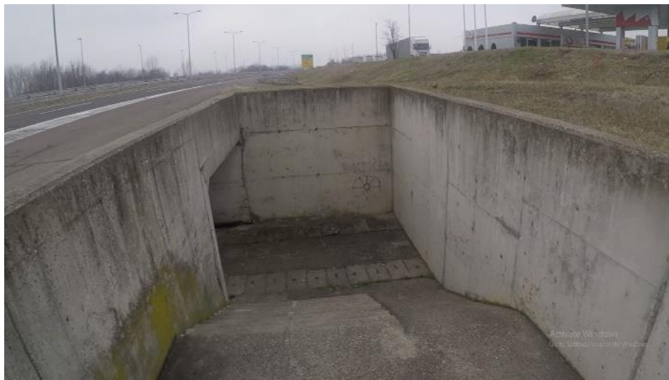
Figure 20. Box culvert for pedestrians
