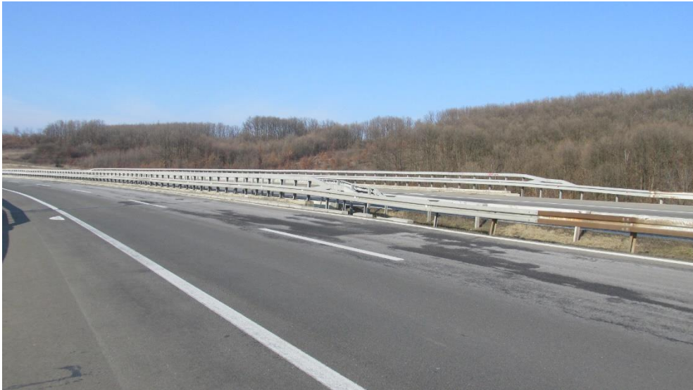
Figure 23. Overpass across the country road at km (Perilovac) at km 383+790
