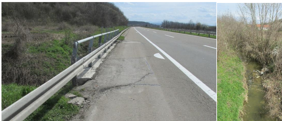
Figure 13. The Bridge over Krezbijski stream at km 367+753
