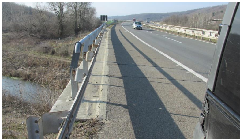
Figure 15. The Bridge over Jovanovacka River at km 375+897
