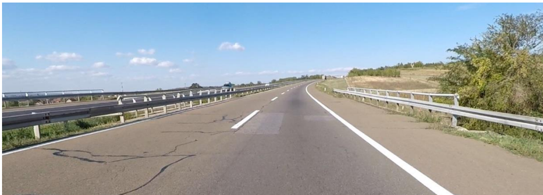
Figure 12. The Bridge over Bacijski stream at km 362+529
