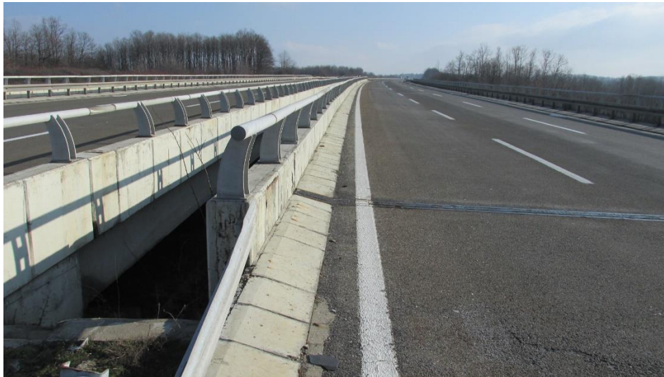
Figure 22. Bracin Viaduct over landslide at km 379+199
