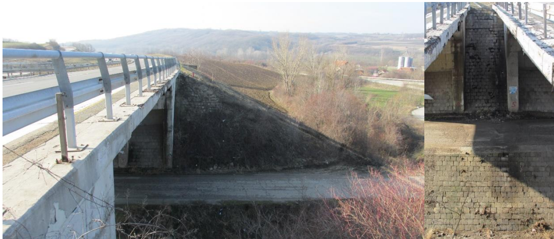
Figure 16. The Bridge over stream and road at km 377+926
