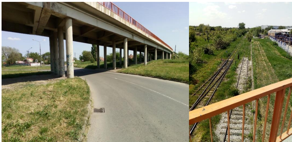
Figure 17. Bekov overpass at ~ km 124+060
