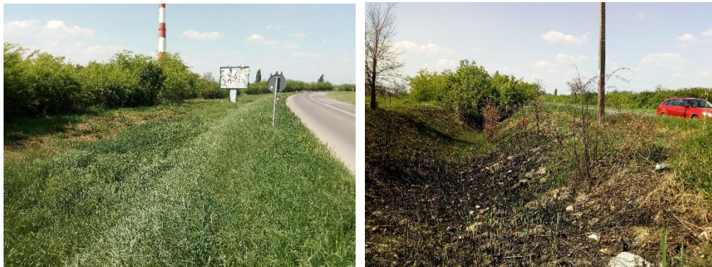
Figure 7. Intake canals on the right side of the road on the subject road section
