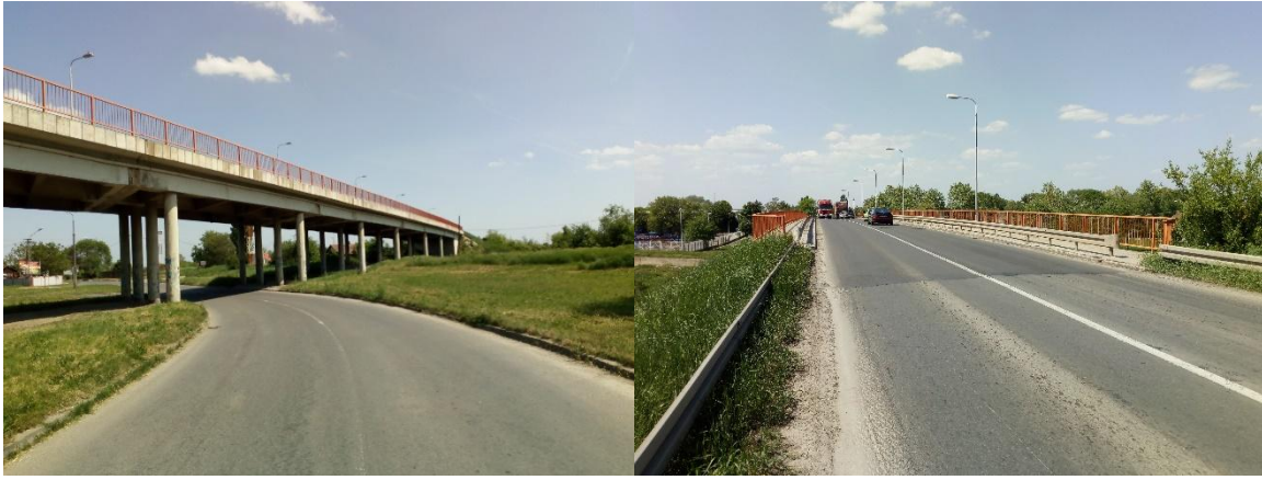
Figure 5. Bekov Overpass at ~ km 124+060
