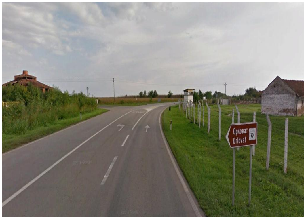
Figure 3. The end of the road section
