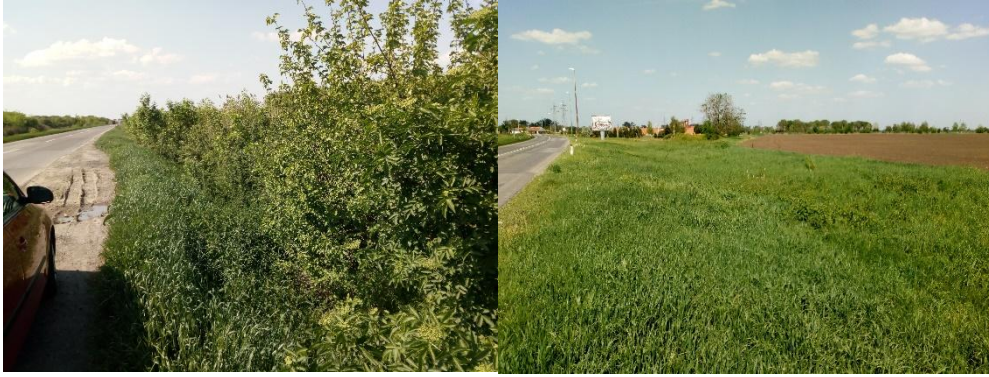
Figure 9. Intake canals on the left side of the road on the subject road section
