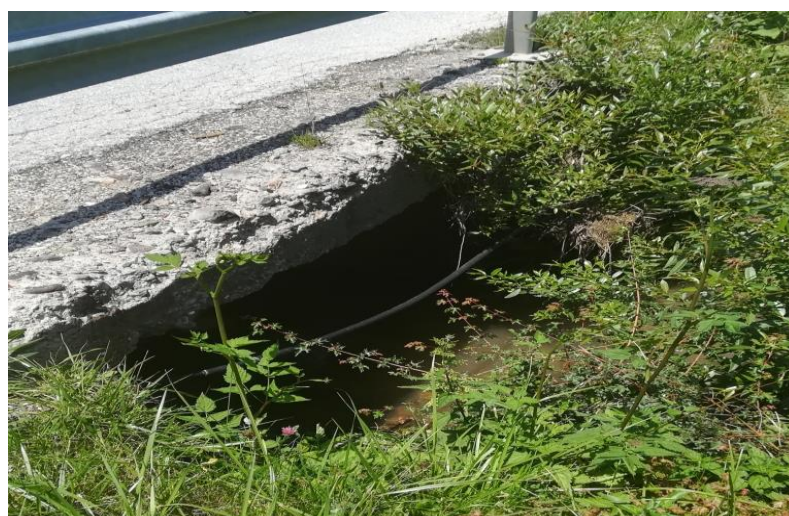
Picture 11. Box culvert on km 90+205.79 (Osaonicki stream)
