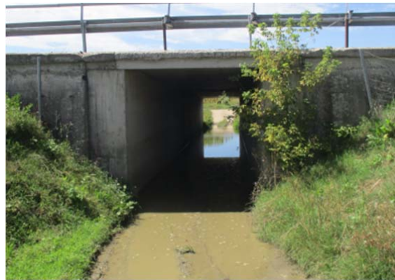
Picture 26 - Box passage at km 451+737
