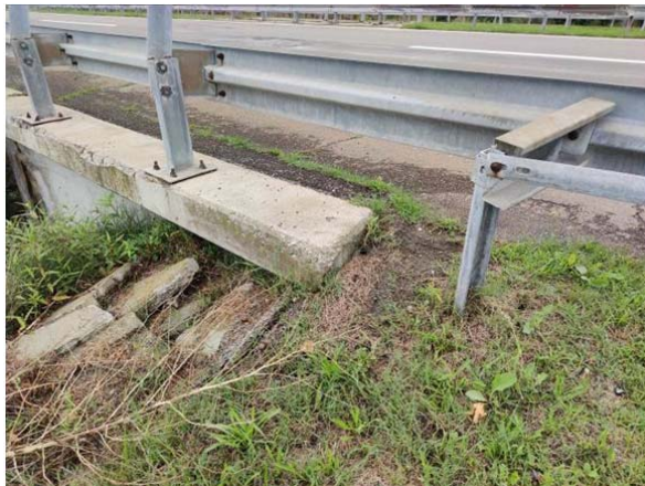
Picture 32- Unchanneled water flow damages the skittles
