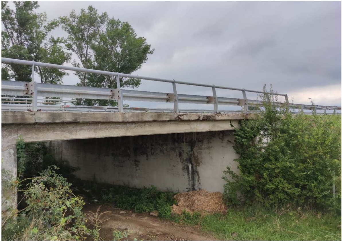
Picture 34- Bottom slopes overgrown by vegetation, unmaintained zone under the bridge, cornices damages
