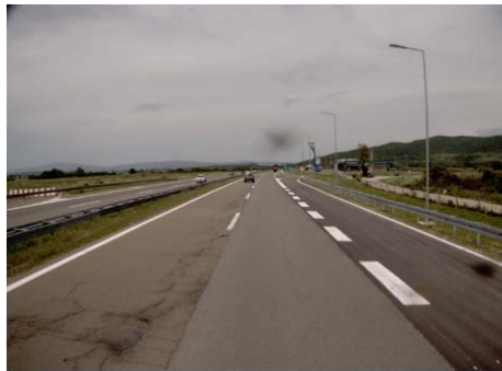
Picture 38. Damage of pavement
