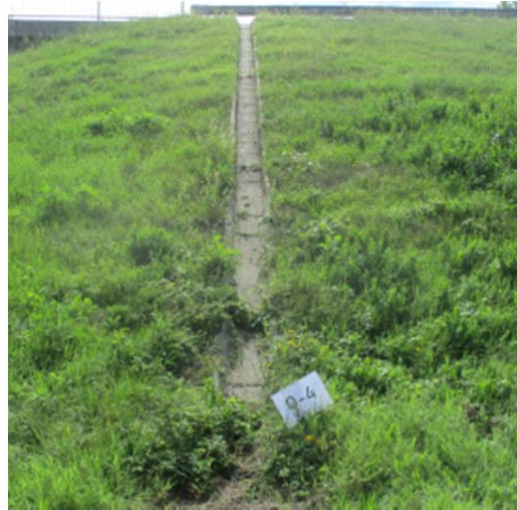
Picture 25 - Typical appearance of the grip condition
