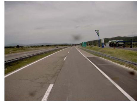
Picture 39. Damage of pavement
