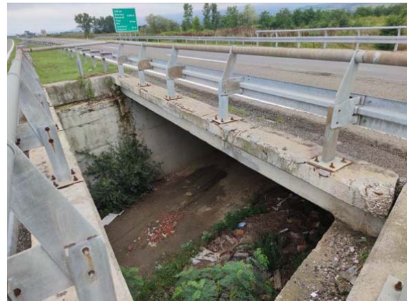
Picture 33- Bridge view in the median
