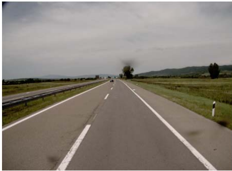
Picture 36. Damage of pavement
