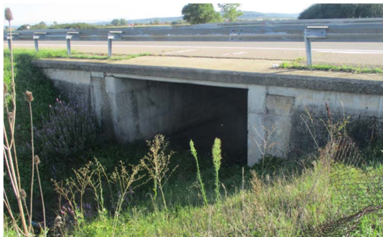
Picture 10 - Box culvert at the station km 454+935
