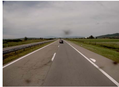
Picture 37. Damage of pavement
