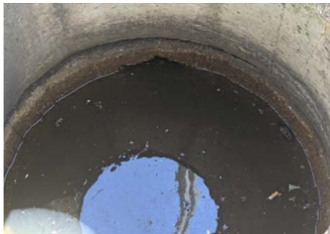
Picture 18 - Water retention in the manhole
