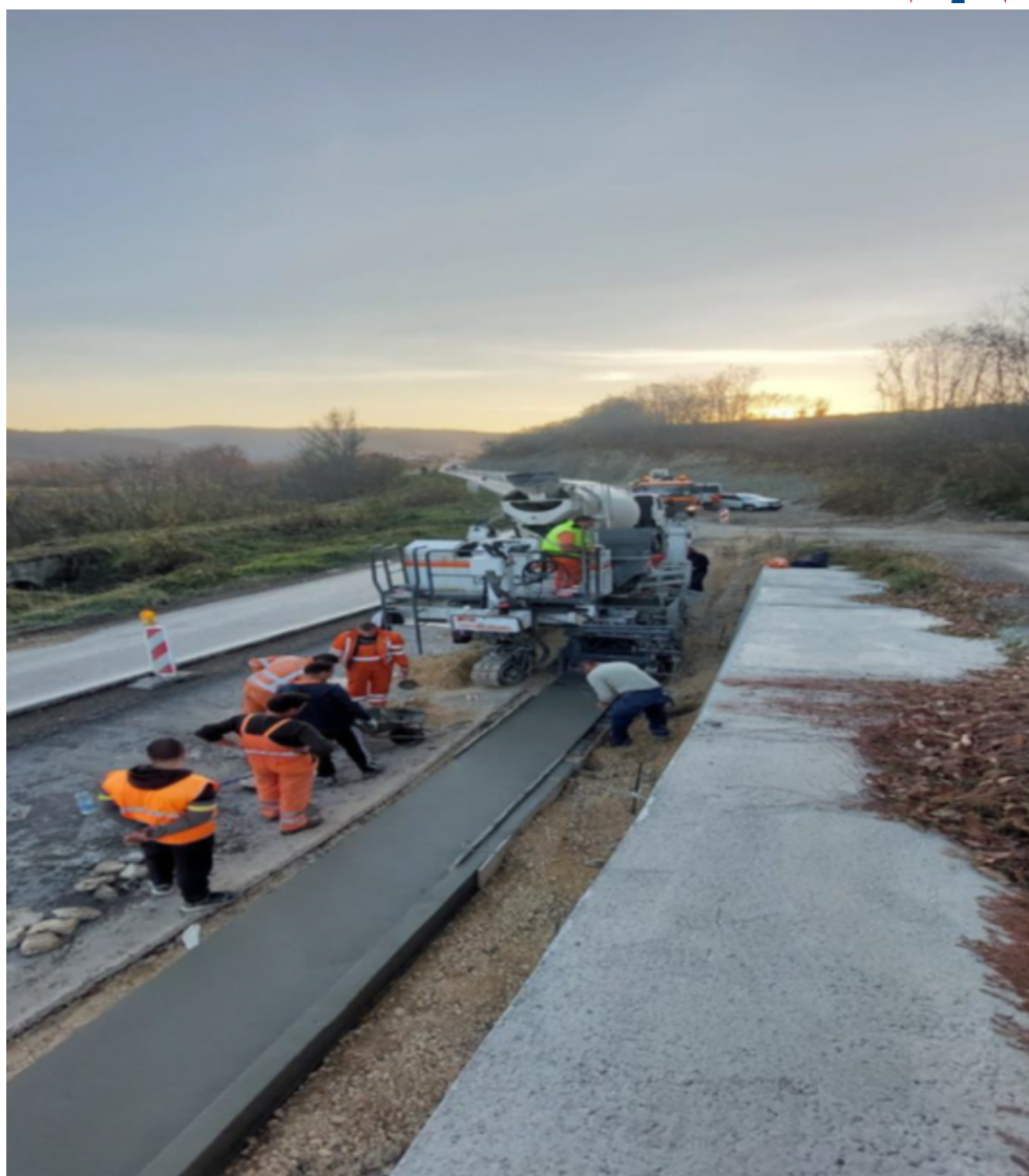
CONSTRUCTION OF GUTTERS
