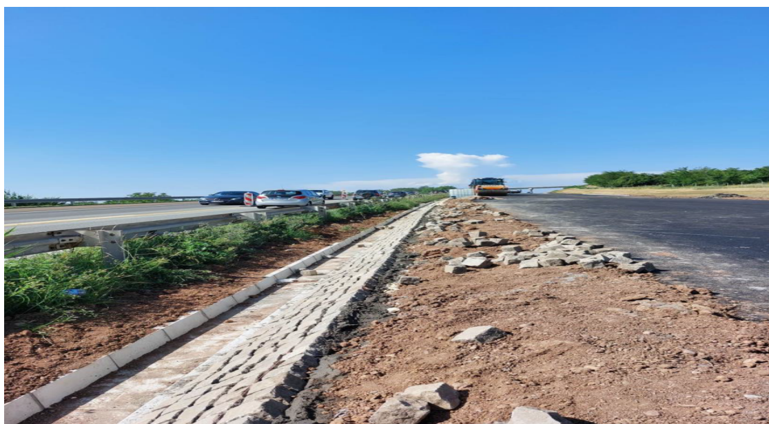
PREPARATION OF THE STONE PAVING ON SLOPES
