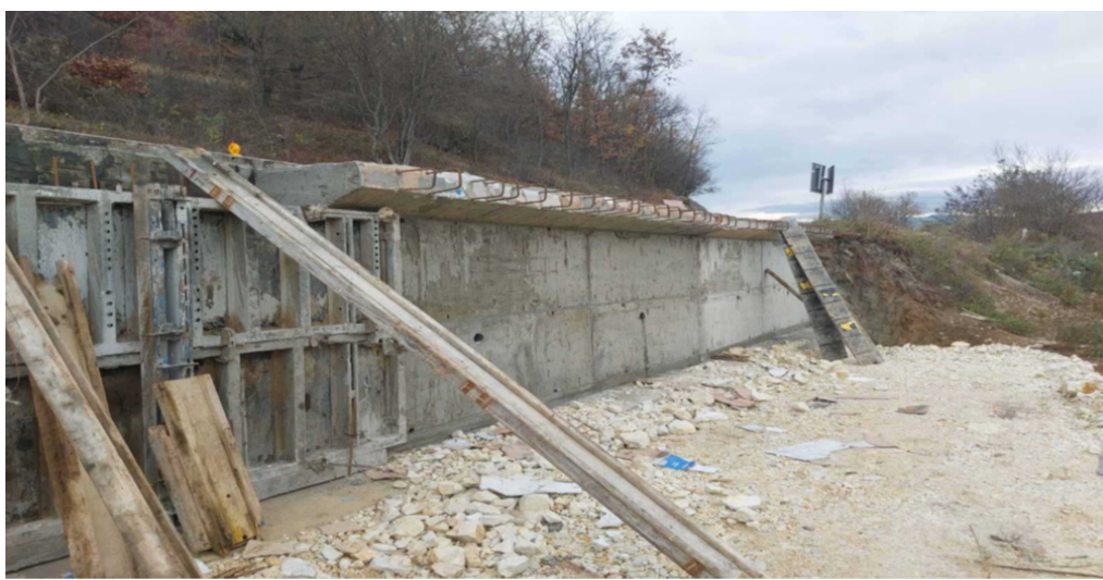
CONSTRUCTION OF AB RETAINING WALLS
