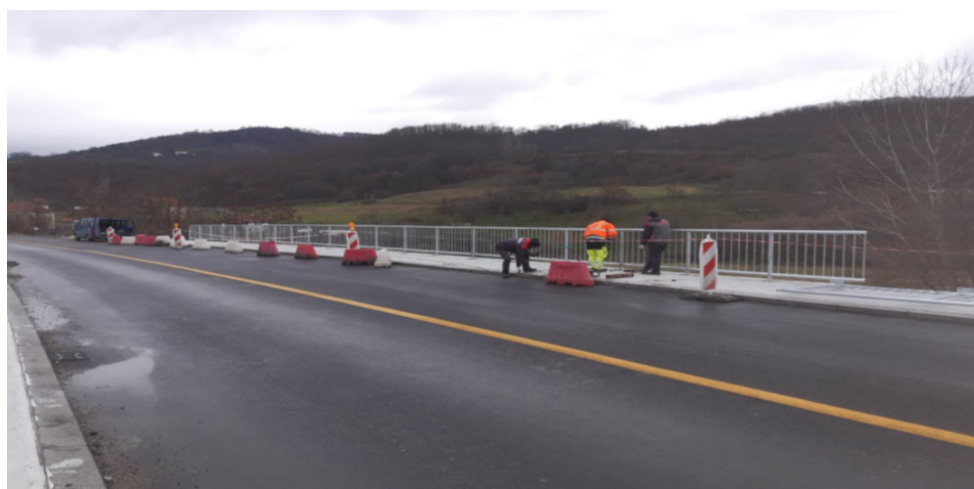
REHABILITATION OF KOSANICA 1 BRIDGE
