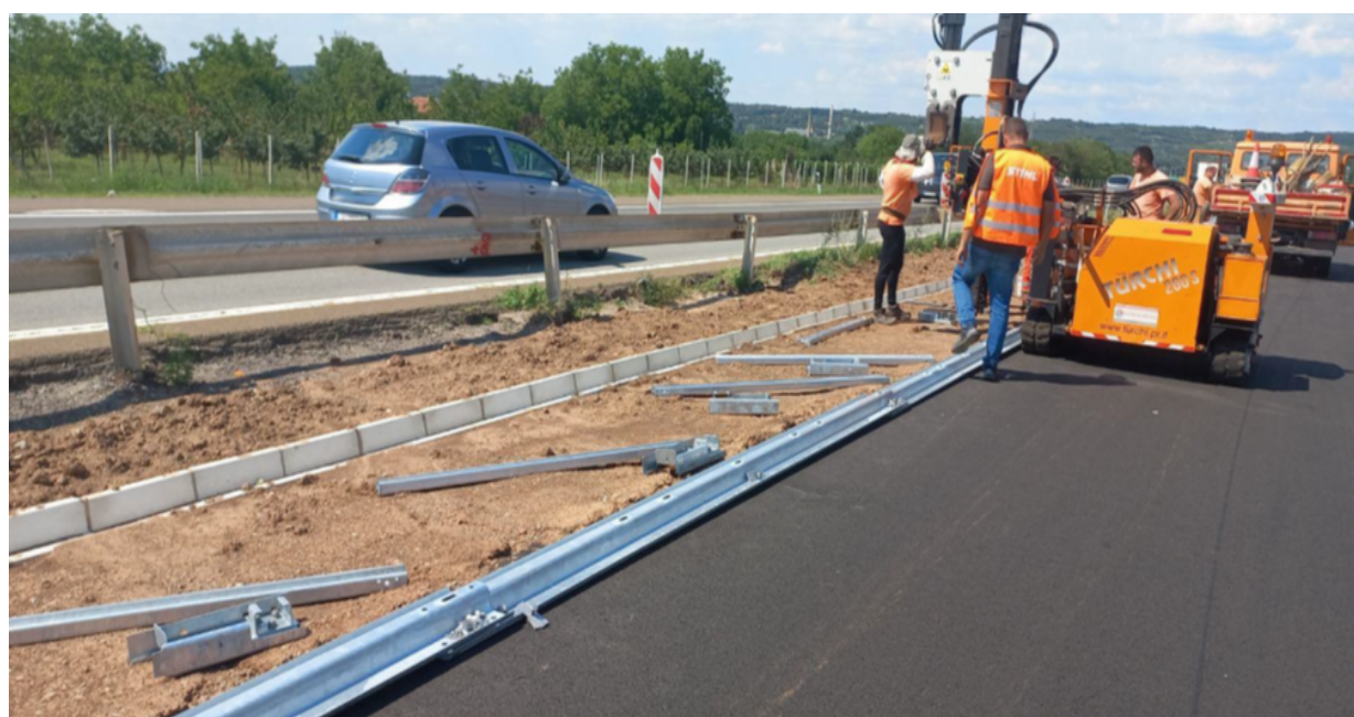
INSTALLATION OF THE FLEXIBLE CRASH BARRIER
