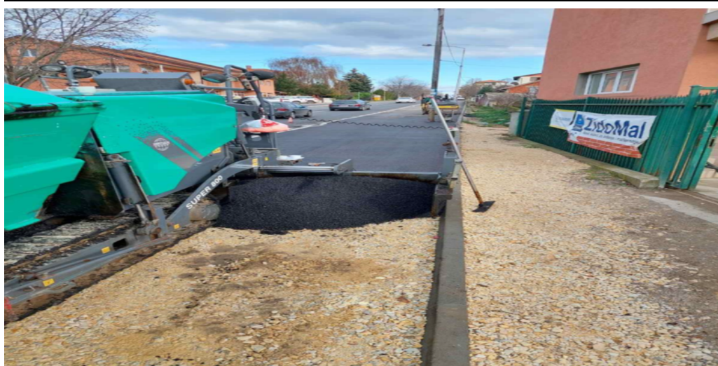
CONSTRUCTION OF PEDESTRIAN FOOTPATHS
