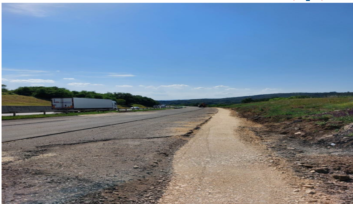
PREPARATION OF THE BASE FOR GUTTER CONSTRUCTION
