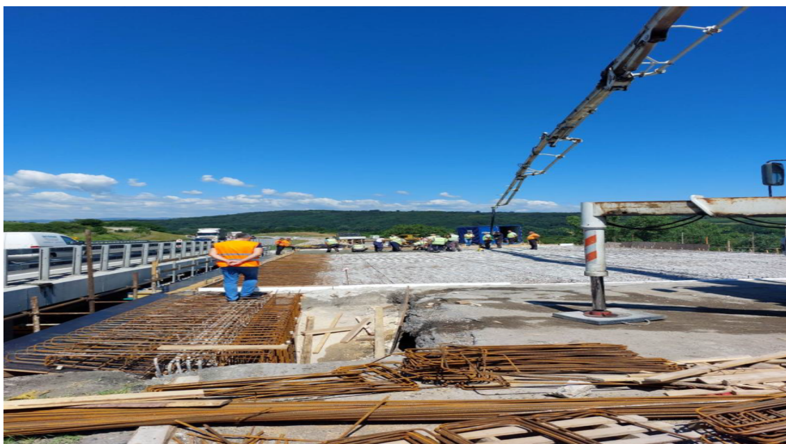
REHABILITATION WORKS ON BRIDGES
