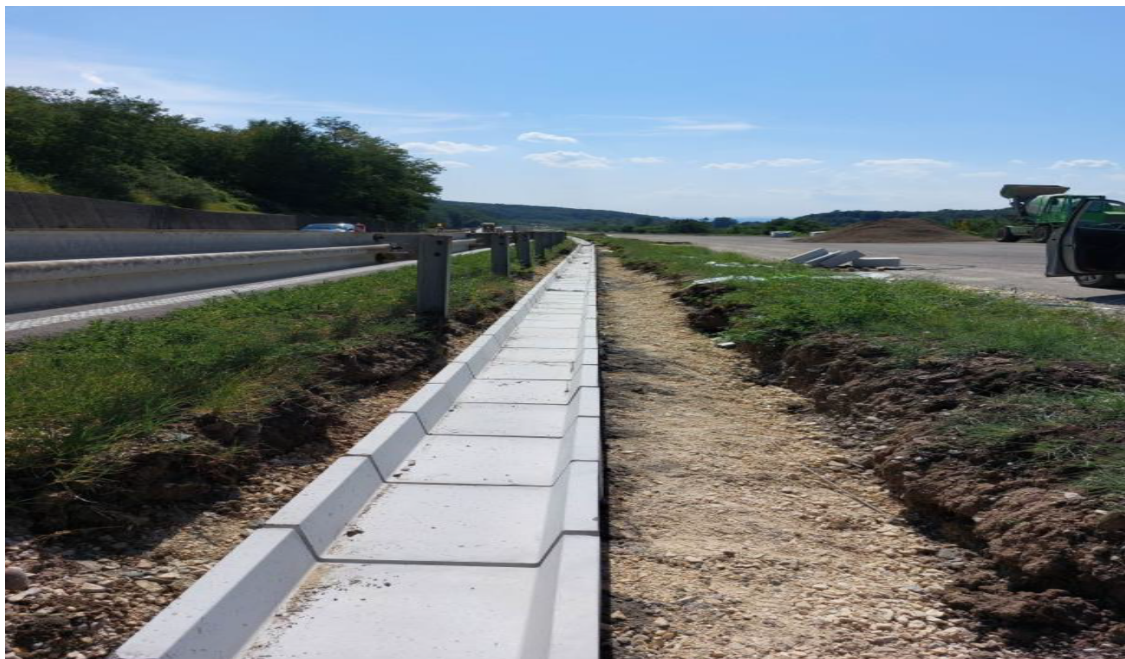
CONSTRUCTION OF DRAINAGE CHANNELS IN THE CENTRAL RESERVATION
