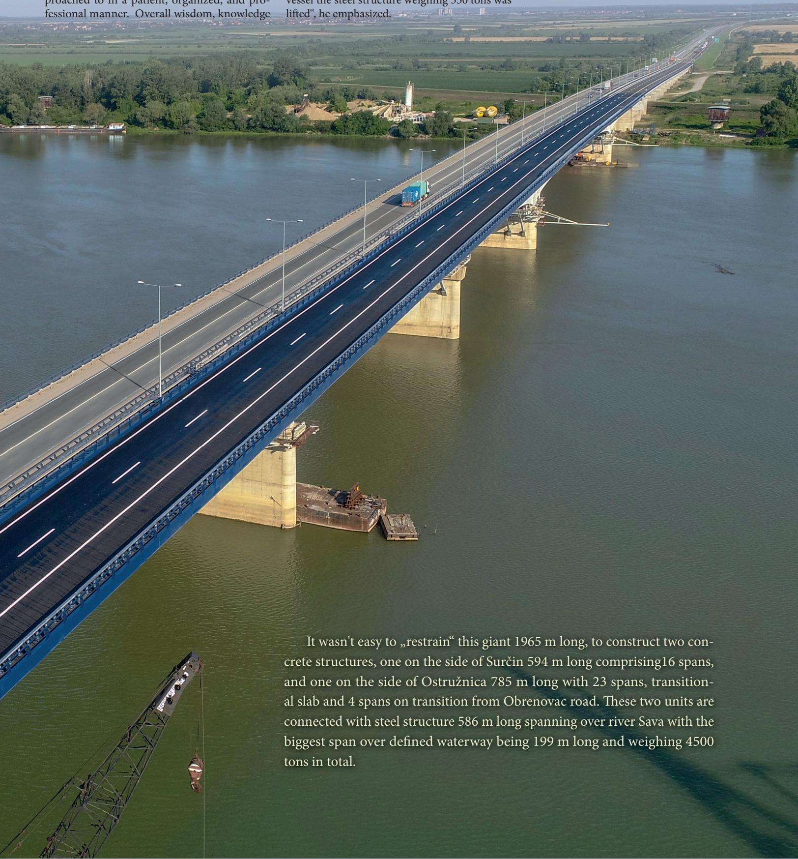
It wasn't easy to „restrain“ this giant 1965 m long, to construct two concrete structures, one on the side of Surčin 594 m long comprising 16 spans, and one on the side of Ostružnica 785 m long with 23 spans, transitional slab and 4 spans on transition from Obrenovac road. These two units are connected with steel structure 586 m long spanning over river Sava with the biggest span over defined waterway being 199 m long and weighing 4500 tons in total.
