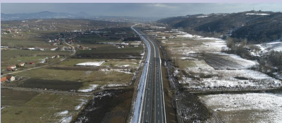
A total of 112.516 tons of asphalt mix was incorporated into this section. For the purpose of foundation of river piers a total of 4.720 meters of piles were constructed, while 6,830 tons of reinforcing and 44.030 cubic meters of concrete were incorporated in bridge structures and overpasses. App. 24.000 linear meters of road fence were placed, and 1.156.000 cubic meters of material was incorporated into the road base .....
