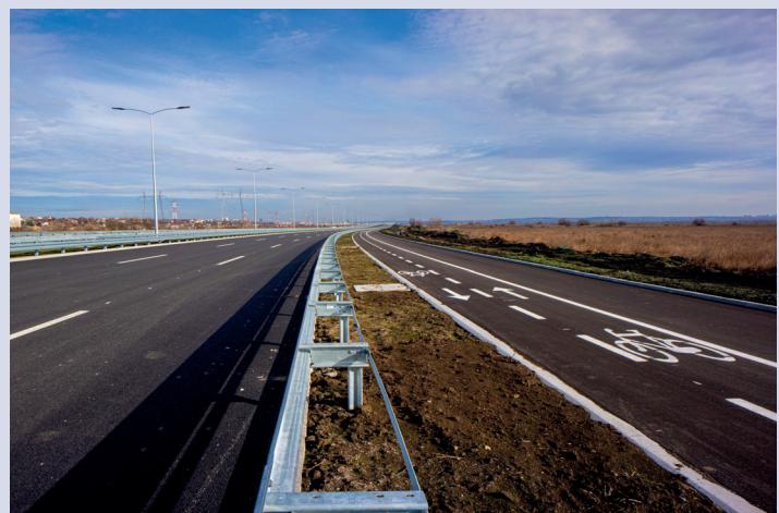
The 7.9km section is designed for a speed of 80km/h and has three 3.5m wide lanes in each direction, a 5m dividing strip, 2m wide pedestrian paths and a 2.2m wide bicycle path. There
