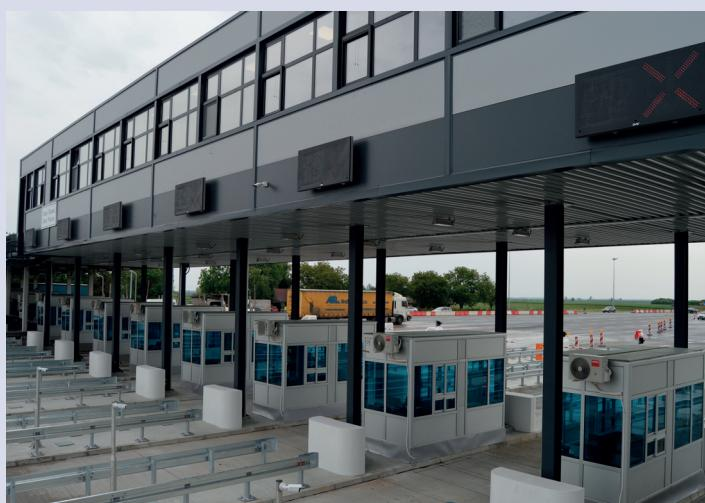
The expansion of the Stara Pazova toll station involved the construction of 8 islands, resulting in a total of 17 traffic lanes, of which at least 3, at any time, are intended exclusively for users of electronic toll collection. Above the toll channels, a modernly equipped administrative building with an area of more than 300m<sup>2</sup> was built. The dimensions of the administrative building, erected 10 meters above the sidewalk of the traffic island, are
