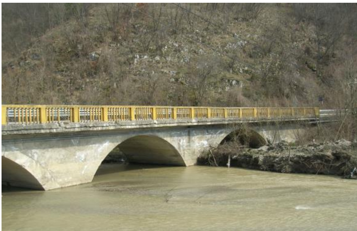
Picture 16. Bridge on the branch of Drina River ~ km 14+680
