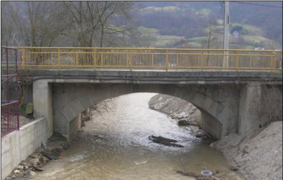
Picture 18. Bridge on the river Velika Reka ~ km 25+474
