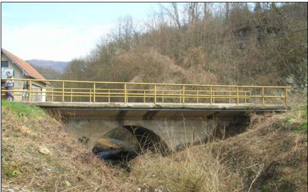
Picture 15. Bridge on the river Pljestanica ~ km 10+527
