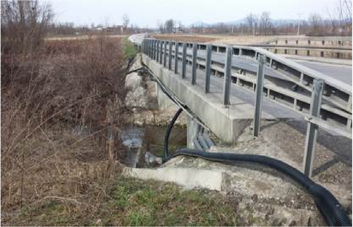
Picture 10: Watercourse at chainage km 6+592 (Lađevci river)
