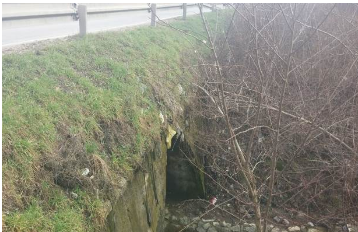
Picture 15: Watercourse at chainage km 10+189 (Đurašinac stream)
