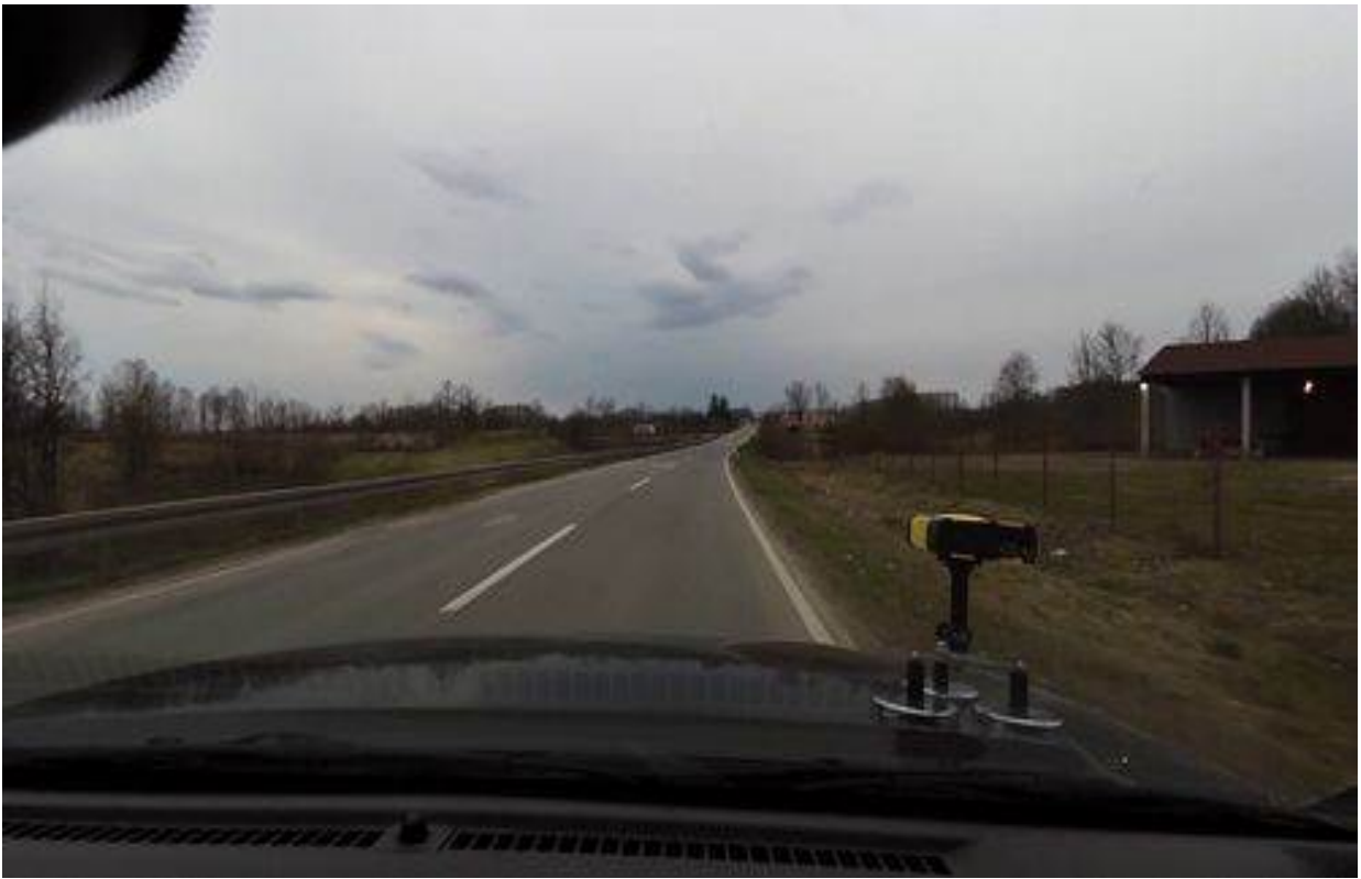
Picture 8: Part of the route on an embankment higher than 3m, on the right as viewed in the chainage growth direction
