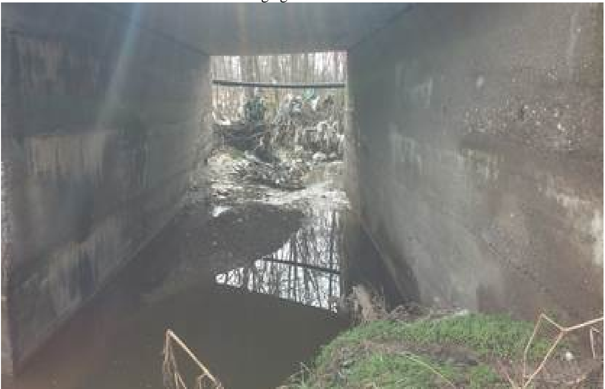
Picture 9: Watercourse at chainage km 6+214 (Bojovac stream)
