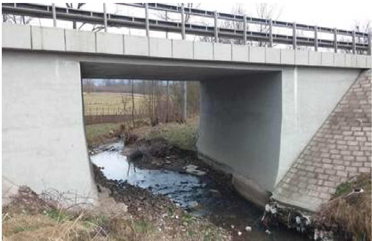
Picture 13: Watercourse at chainage km 8+180 (Bubanj stream)
