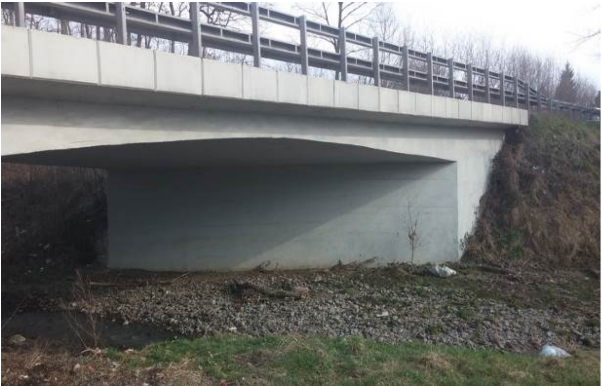
Picture 17: Watercourse at chainage km 11+050 (Gradinac stream)
