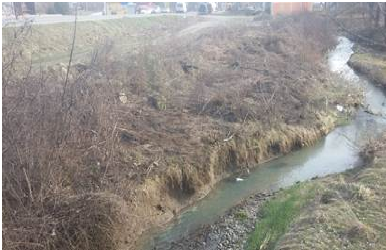
Picture 18: Watercourse at chainage km 11+330 (embankment fortification in Miločaj)
