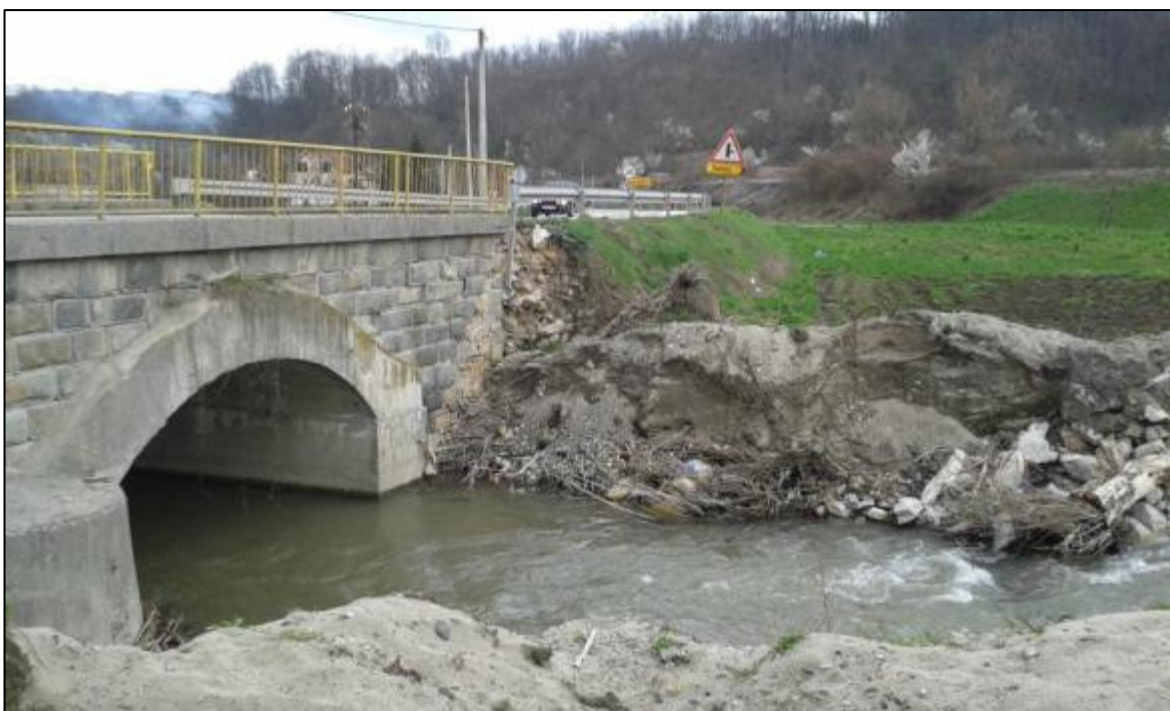
Picture 9. Bridge over the Radaljska River ~ km 12 + 265
