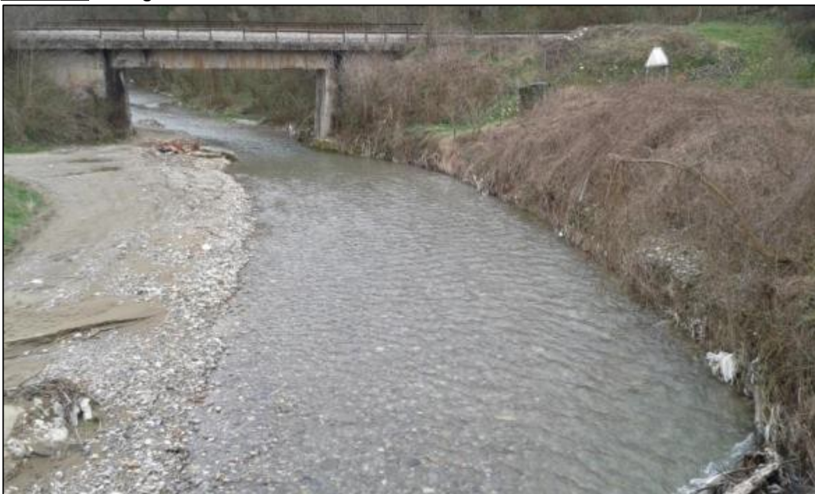
Picture 8. Bridge over the Borinska River ~ km 9 + 130
