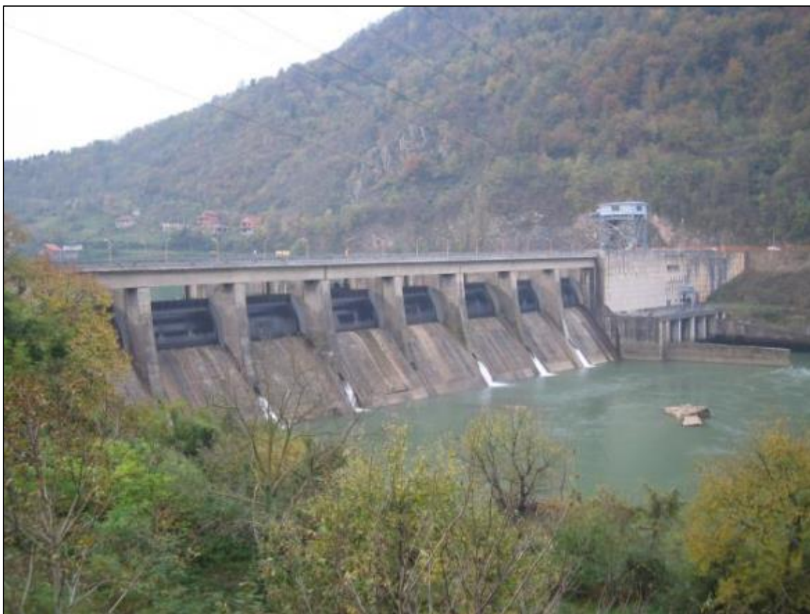
Picture 10. Hydroelectric power plant "Zvornik"
